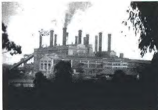
YALLOURN POWER STATION
