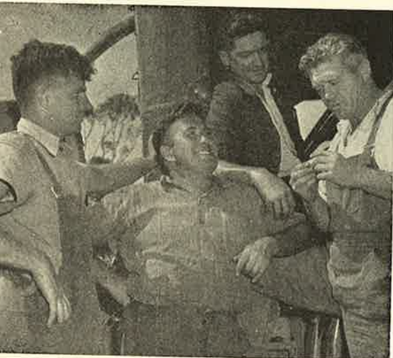
Waiting to follow the dredger over the river are drivers of the trucks carrying 6,000 yards of high tension cable: John O'Connell, Sam Rothsay, Peter Shann. Mechanic Bert Spokes in cabin.
