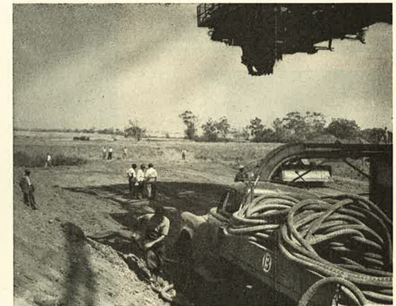
Any moment now . . . the causeway is ready; cable trucks stand by.
