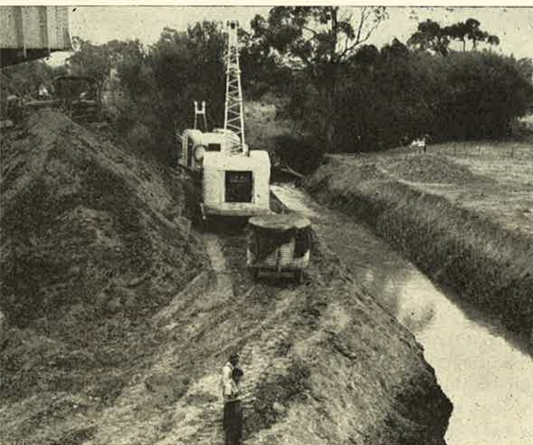
Looking from the dredger along the temporary river channel.
