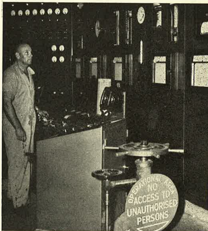
Fireman Harold Atkinson keeps a close watch on the indicators of No. 8 boiler control. Feeding the boilers is carefully controlled. ▶
