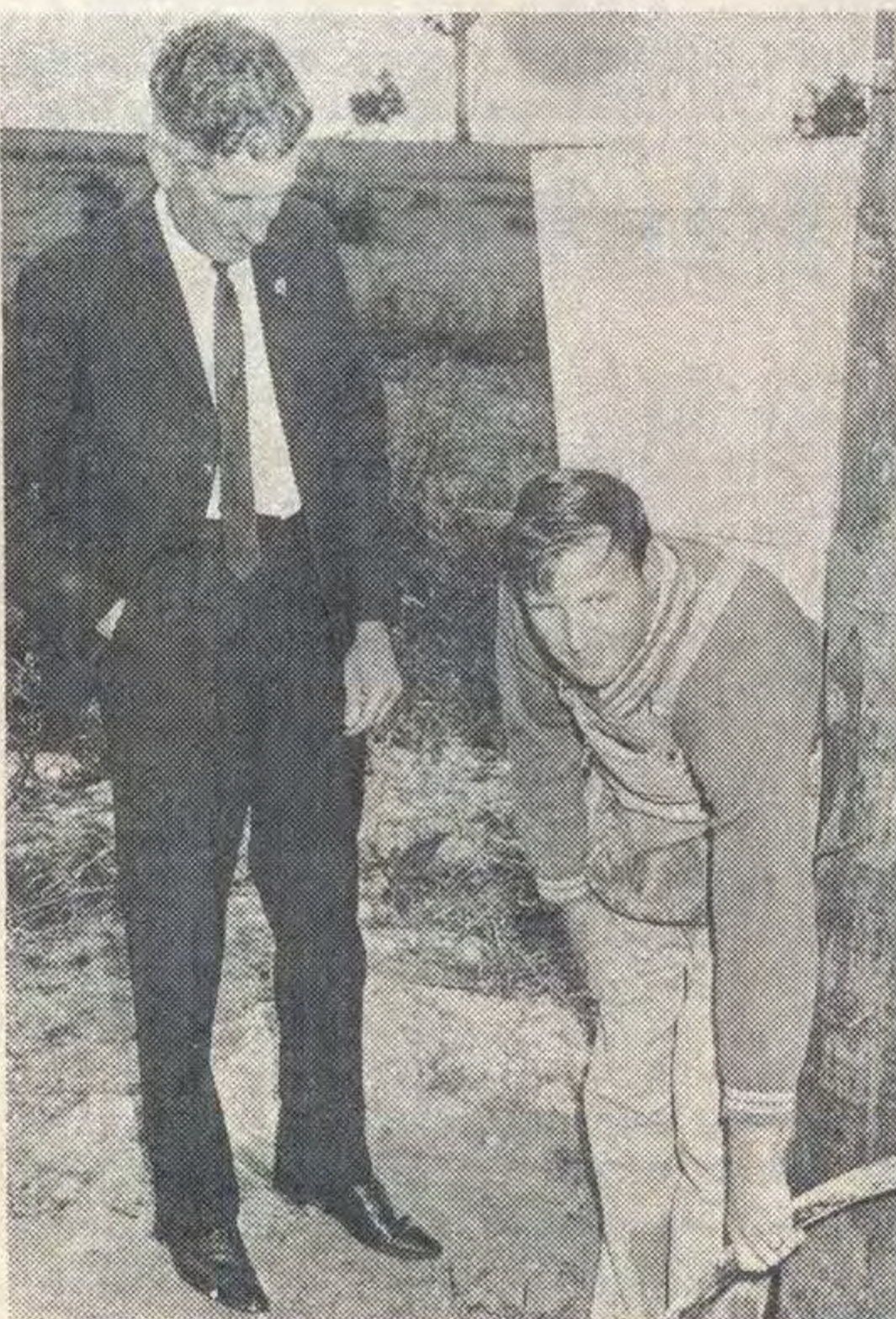
• REGION'S representative on the Aquatic Centre committee, Mr. Tom Stillman (Gen. Services Supt. Morwell) pictured with Petch Constructions (Trafalgar) carpenter Ken Bechaz during construction last week.
