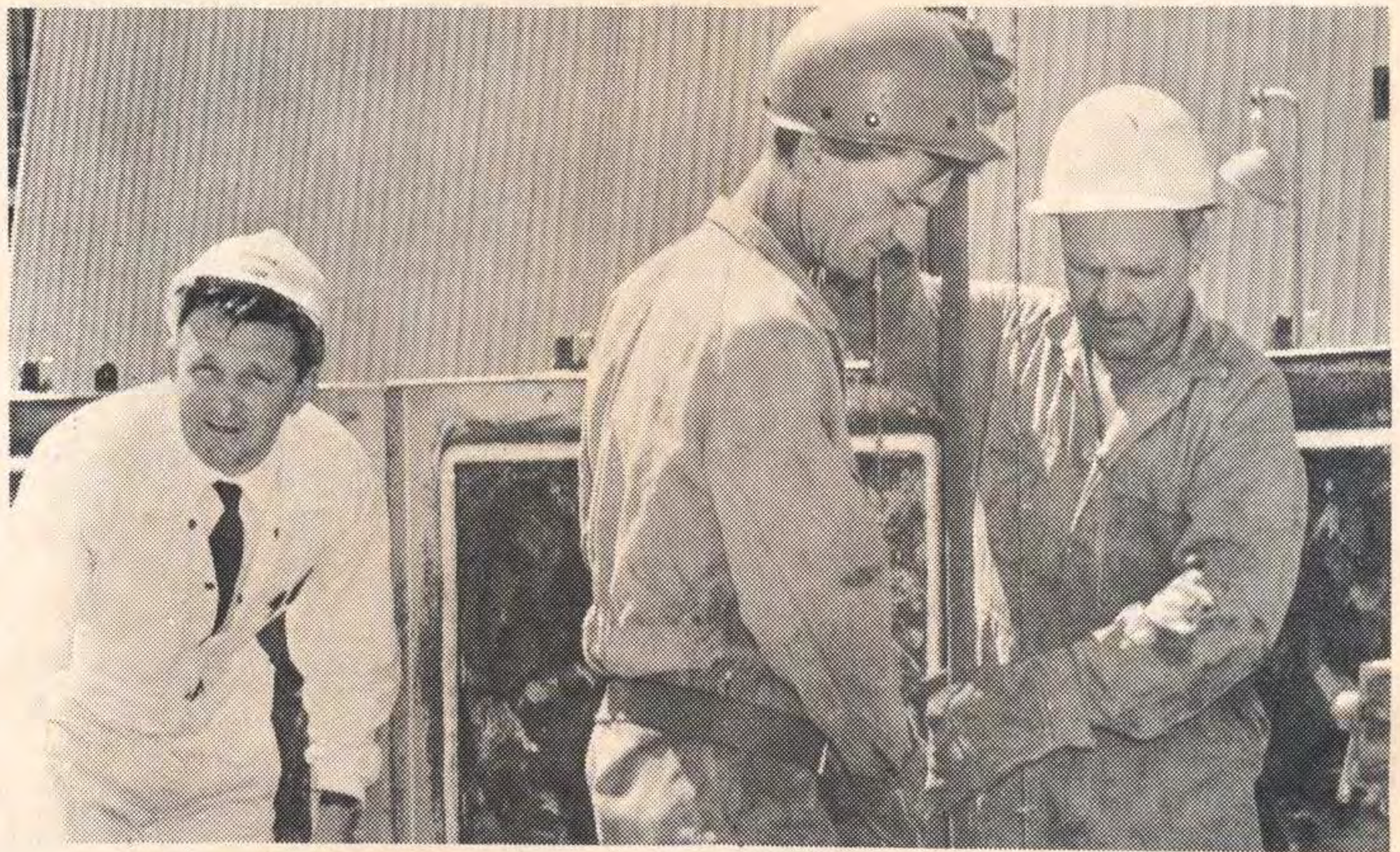
* REMOVING steel rods from the roof of a precipitator are riggers M. Lions and A. Mifsud. Foreman Stan Randall is at left.
