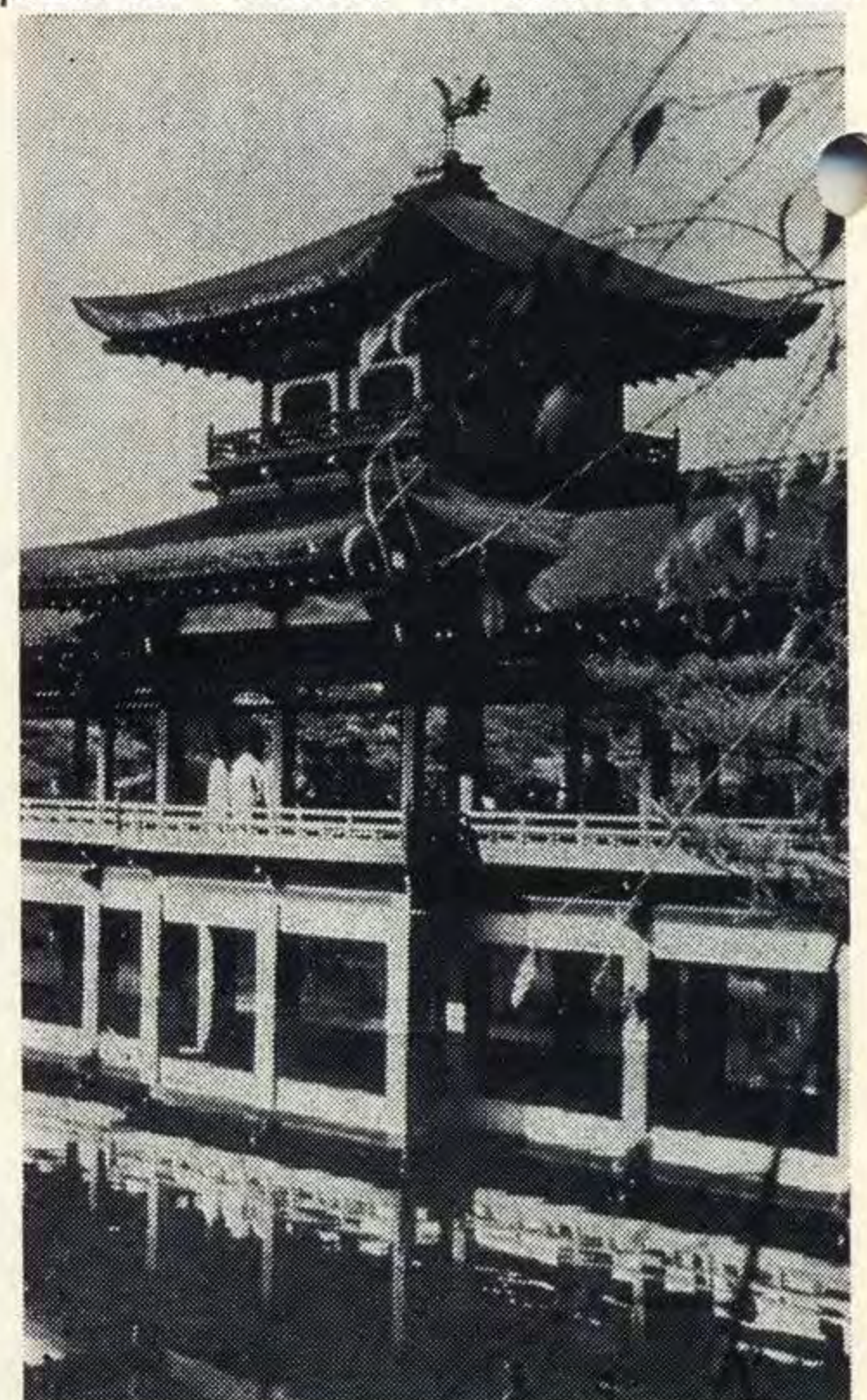
Bridge over a pond at the Heian Jingu Shrine.
