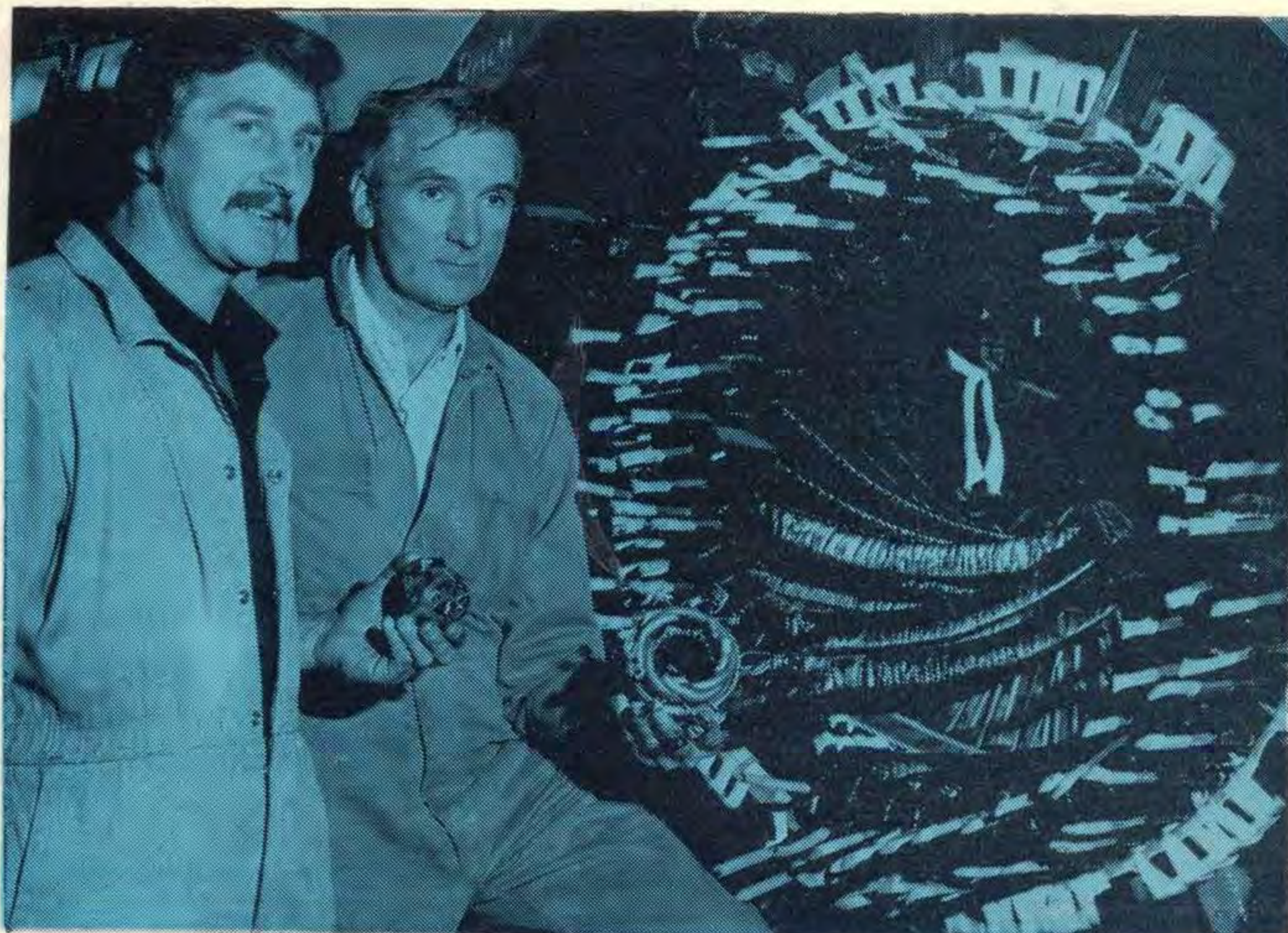
Leading Hand Electrical Fitter Ken Downs and Armature Winder Fred Jobson holding small motor stators—a big contrast to the 2,900 h.p. boiler feed pump motor stator from Hazelwood Power Station in the background.
