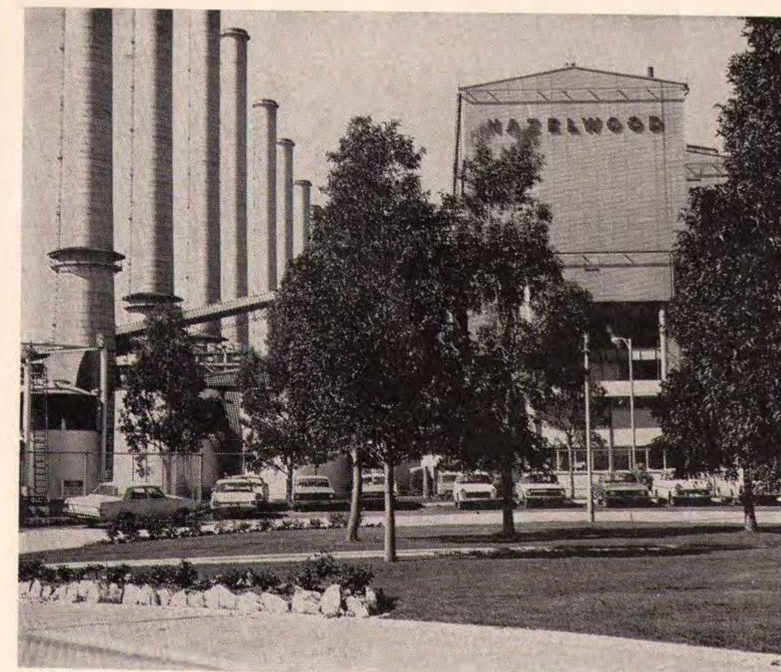
Tall trees and rockery plants frame the station at the south entrance
