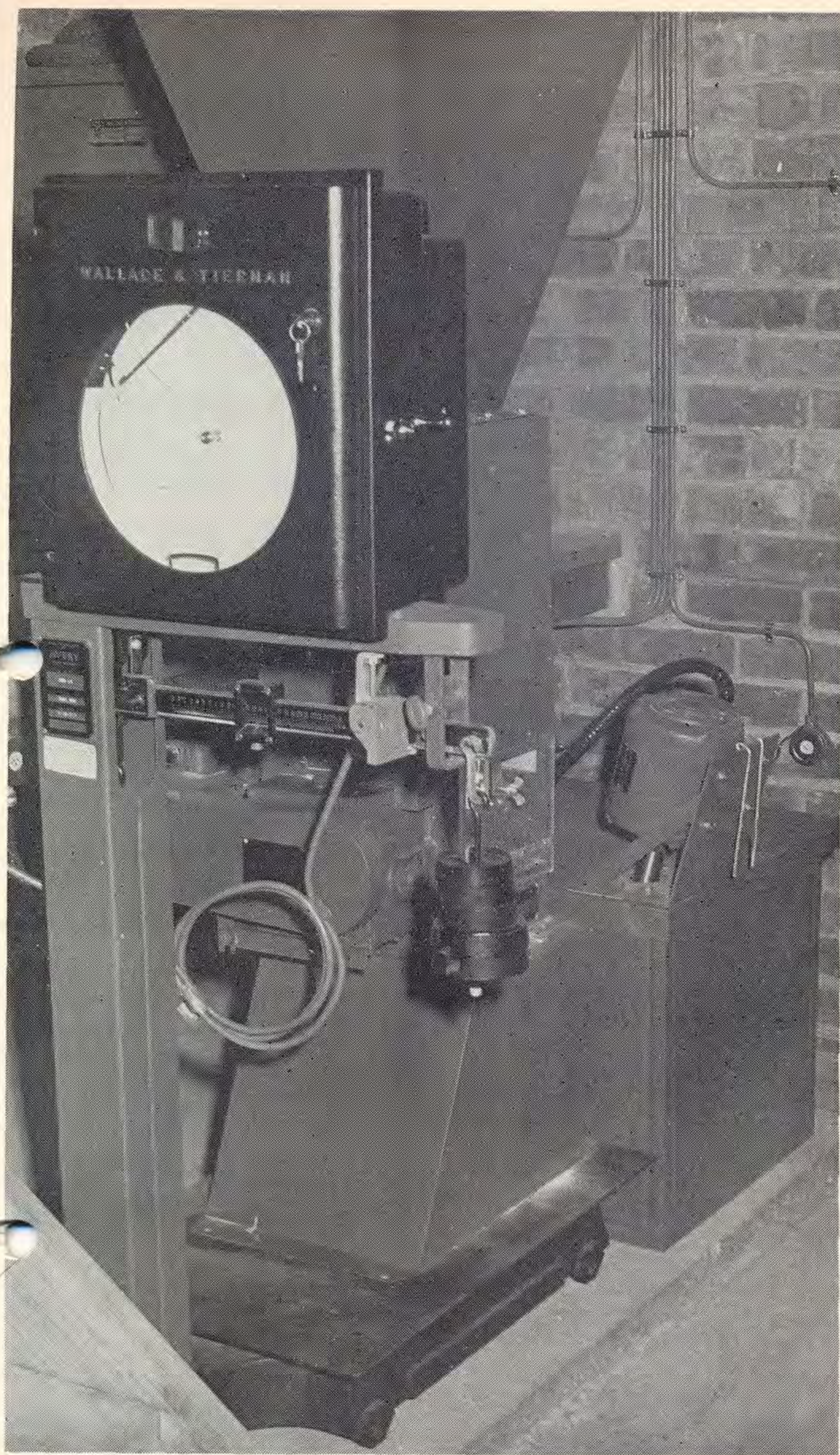
Heart of the fluoridation equipment—the hopper, mixer and loss of weight recorder.
