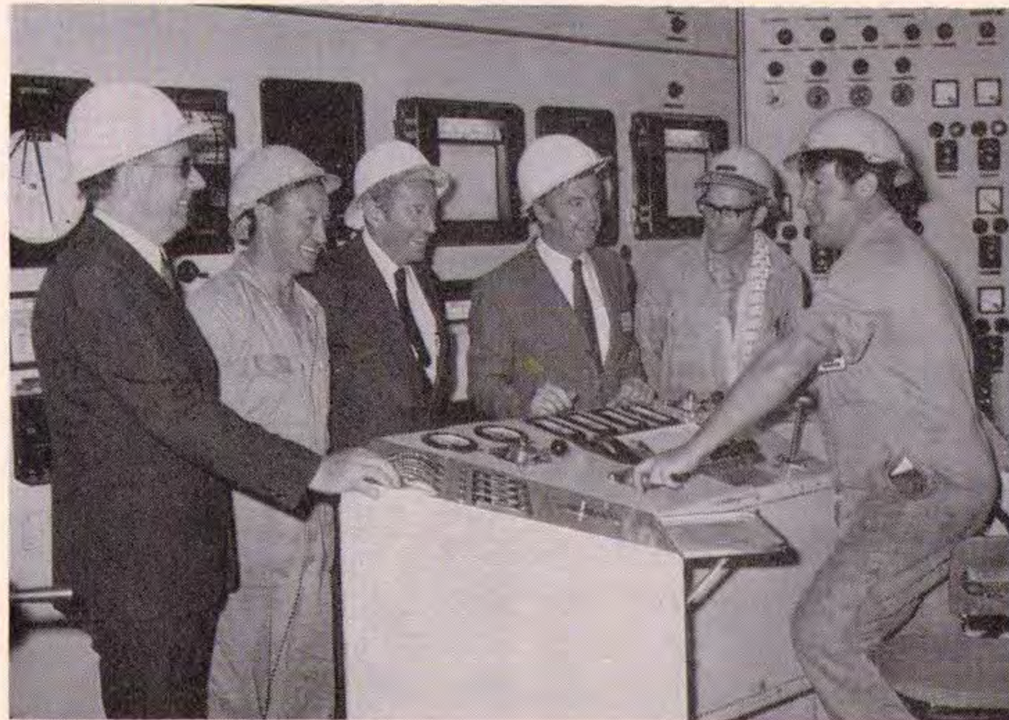
Regulating Fireman John Robinson at the controls of D1 Boiler, Yallourn Power Station, gives the good oil to (left to right) S.E.C. Secretary Frank Chipperfield, L/Fireman Keith Slade, Sir Roger Darvall, Deputy General Manager Charles Trethowan and L/Fireman Athol Jones.
