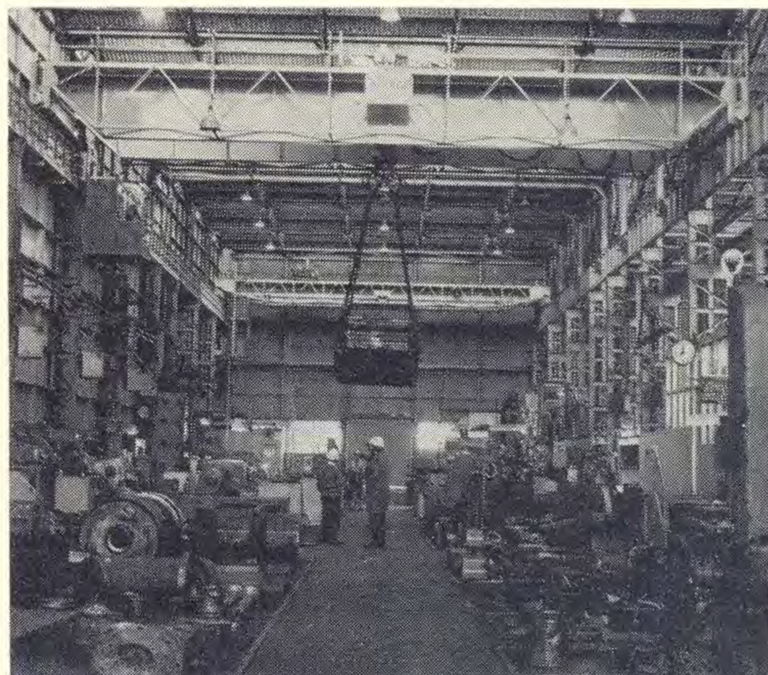
With safety uppermost in mind the entire machine bay was cleared for the downshop travel test using a full load of 50 tons.
