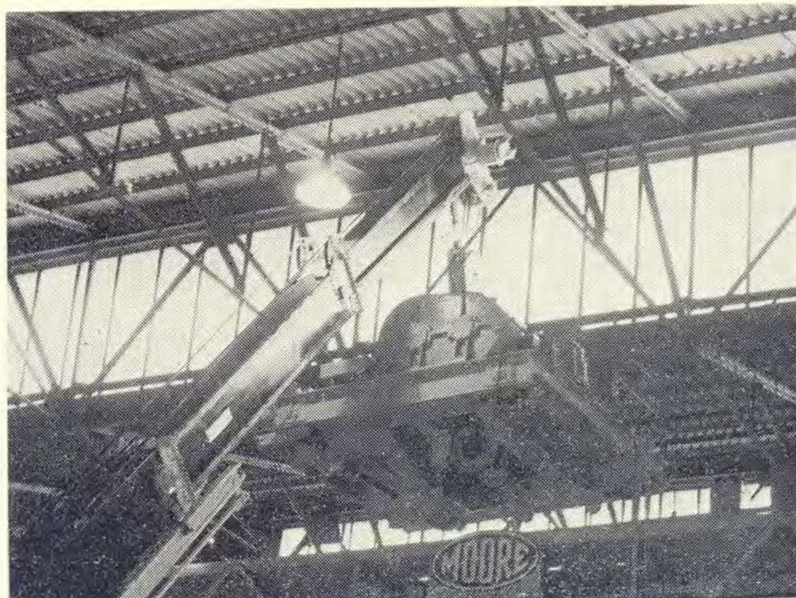
With the jib head almost touching the roof the winch unit is ready to be lowered onto the bridge girders.
