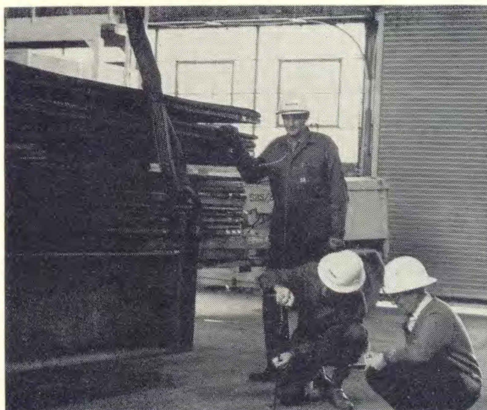
Rigger Bob Wade stands by the load as Civil and Architectural Dept. Engineers Brian Clements and Albert Walker measure the bridge girder deflection.
