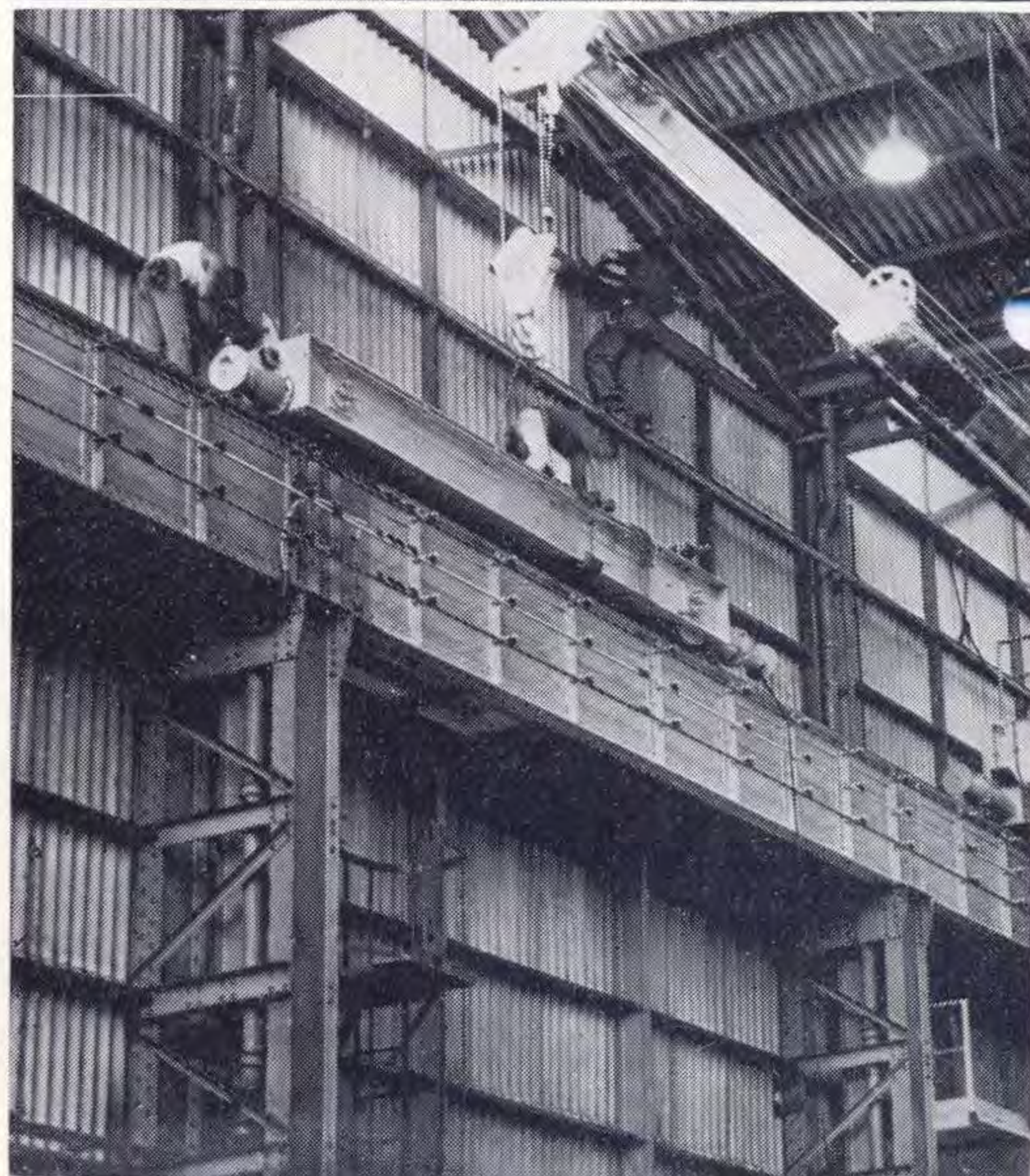
The first end carriage is secured onto the crane rail—note the boom of the mobile crane which can jib out and hoist simultaneously.
