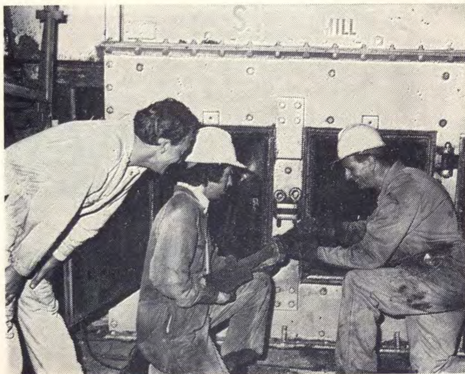
Dennis Buckley (Acting Overseer), Dennis Sealy (apprentice) and Harry Shillinglaw (Trades Assistant) at the restoration of hammer arms of a main pulverising mill of a boiler.
