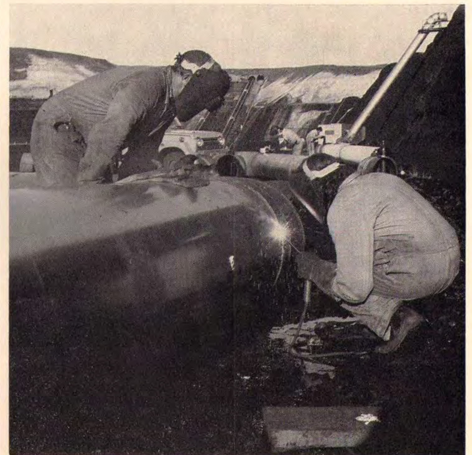
T.A. Dave Mildenhall and apprentice boilermaker Ian Holmes of Morwell Workshops weld up steel pipes inside the open cut.
