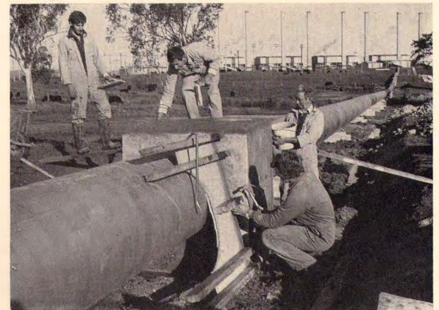
Morwell Civil Works men, from left to right, Bruno Spehar, plasterer; Phil Potter and Ron Martin, builder's labourers, and Peter Lindlow, carpenter, working on an anchor block as part of the 30in. diameter pipeline to the Hazelwood Pond.
