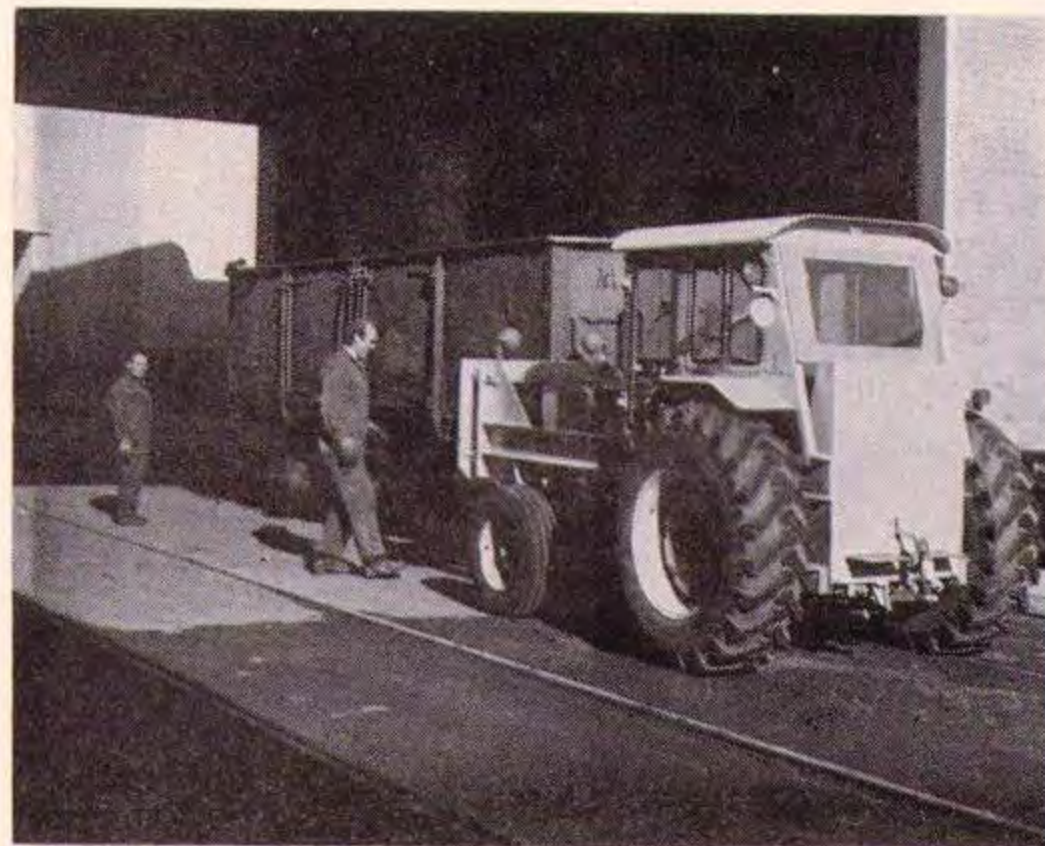
Here we see a truck carrying the ordered items being moved into position prior to unloading. Directing the operation are Leading Hand Rigger Arie Winkelman and Rigger Jan Maciejewski. The items are then unloaded.
