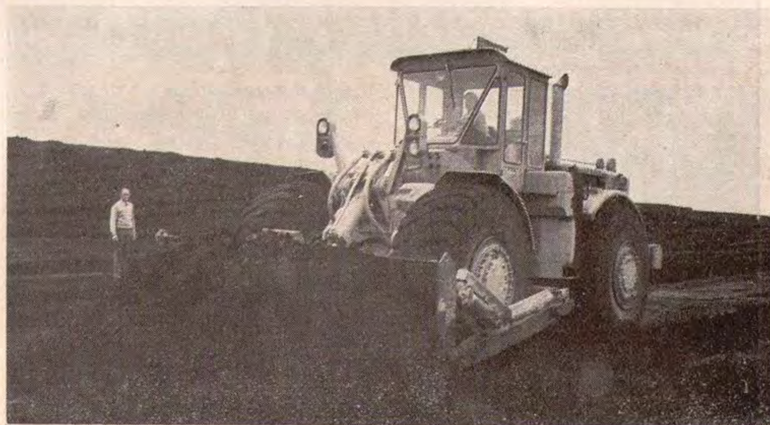
Jack Carter had one of the most important jobs associated with the No. 12 dredger—preparation of the construction site and of ramps and pathways for travel to the open cut.
