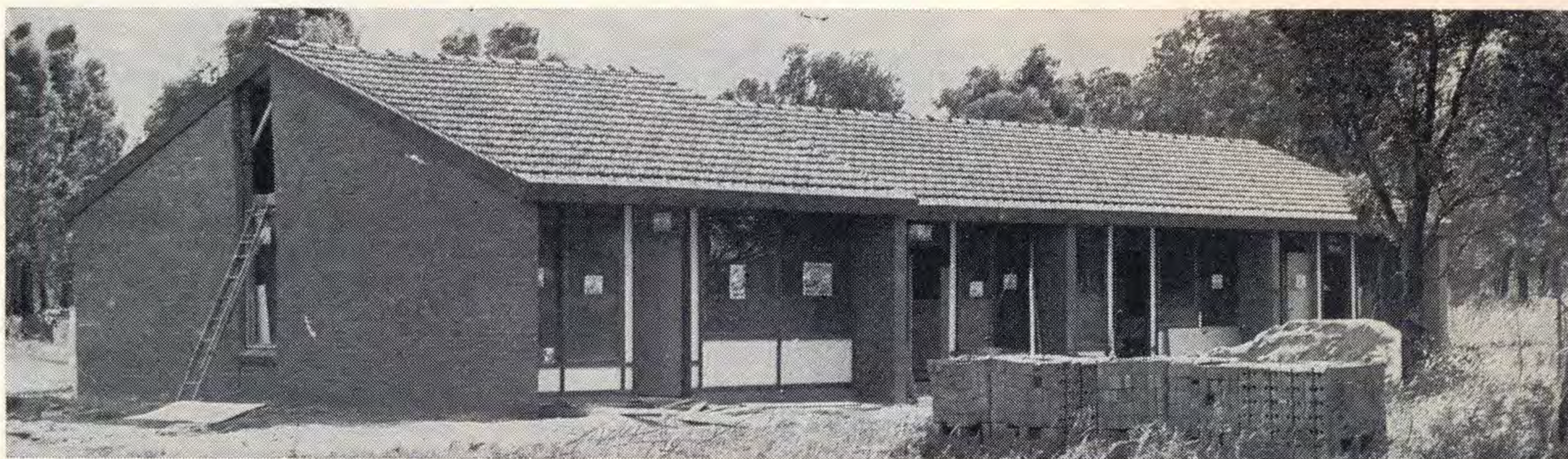
Above: Elderly citizens' flats in the Latrobe Valley Village for Senior Citizens at Newborough (behind the LV Community Hospital) near completion.
