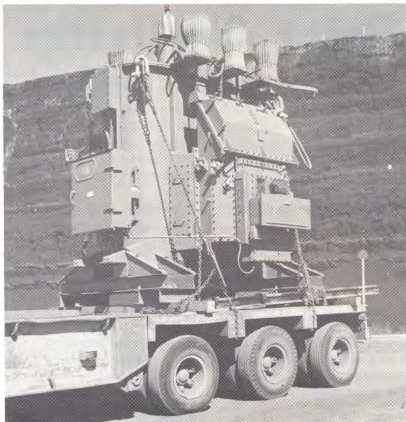
Pictured en route to the new Yallourn YC sub-station is one of the 25 ton transformers from Yallourn YS.
