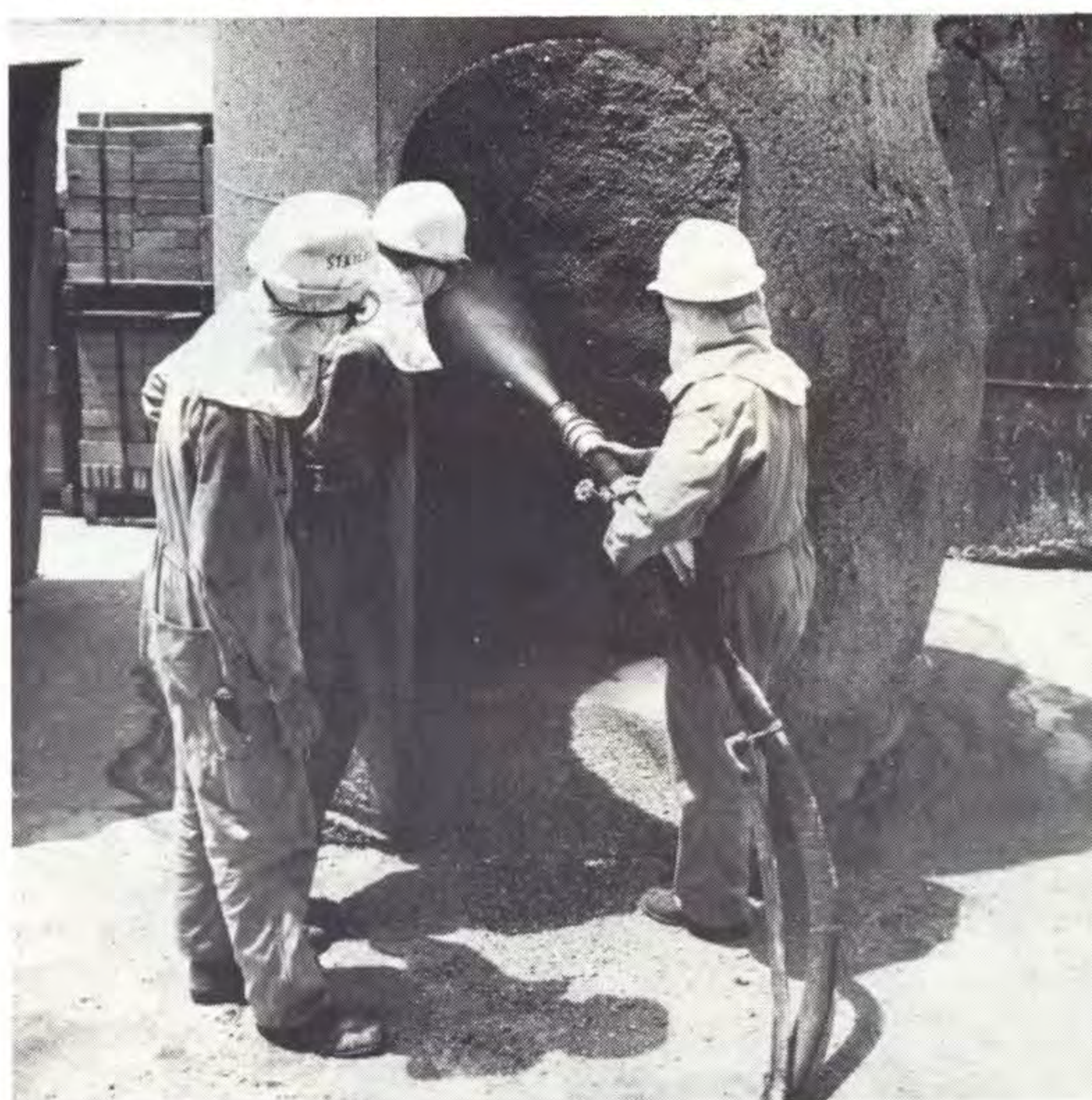
Pictured above during the recent school held at Yallourn on Guniting are (from left), John Bowyer, Geoff Knowles and leading hand bricklayer John Kingsley.
