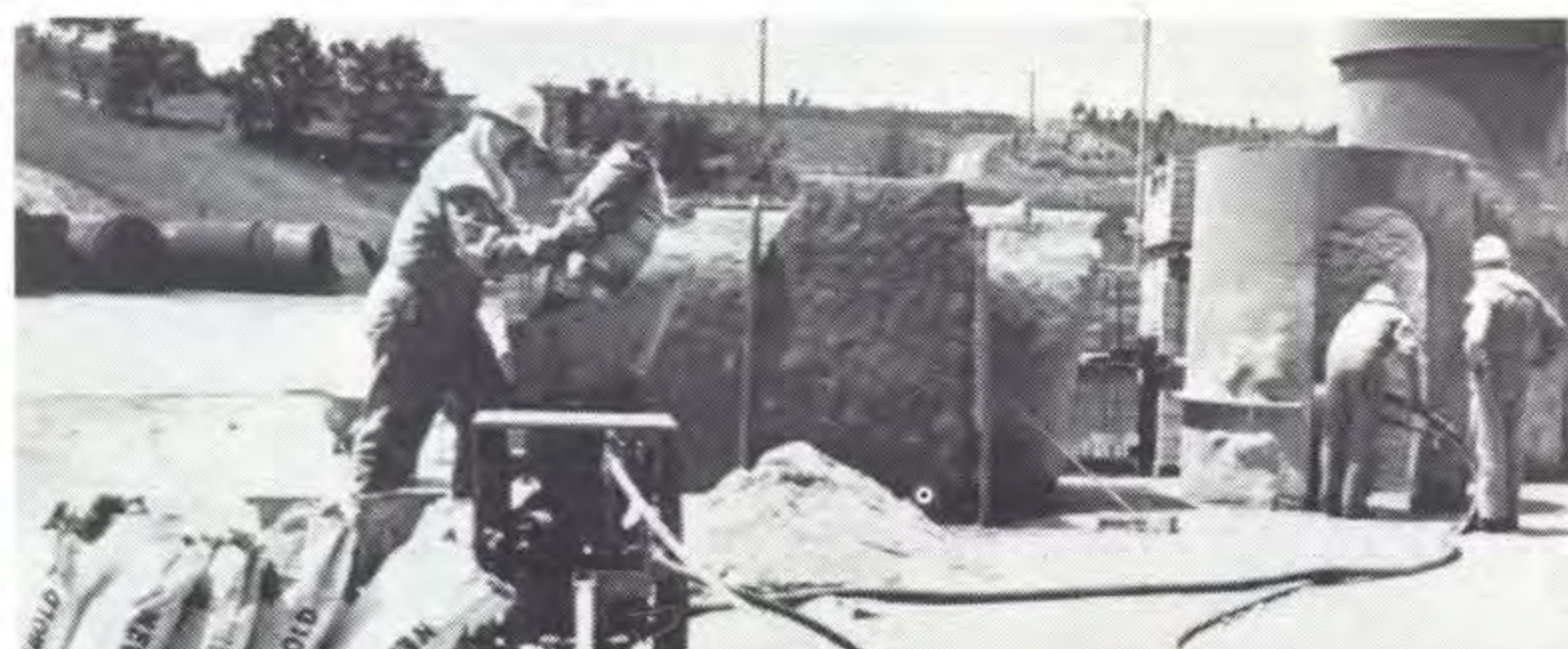
A special model power spray is used to apply the gunite. Pictured above are Commission employees working with the guniting process.
