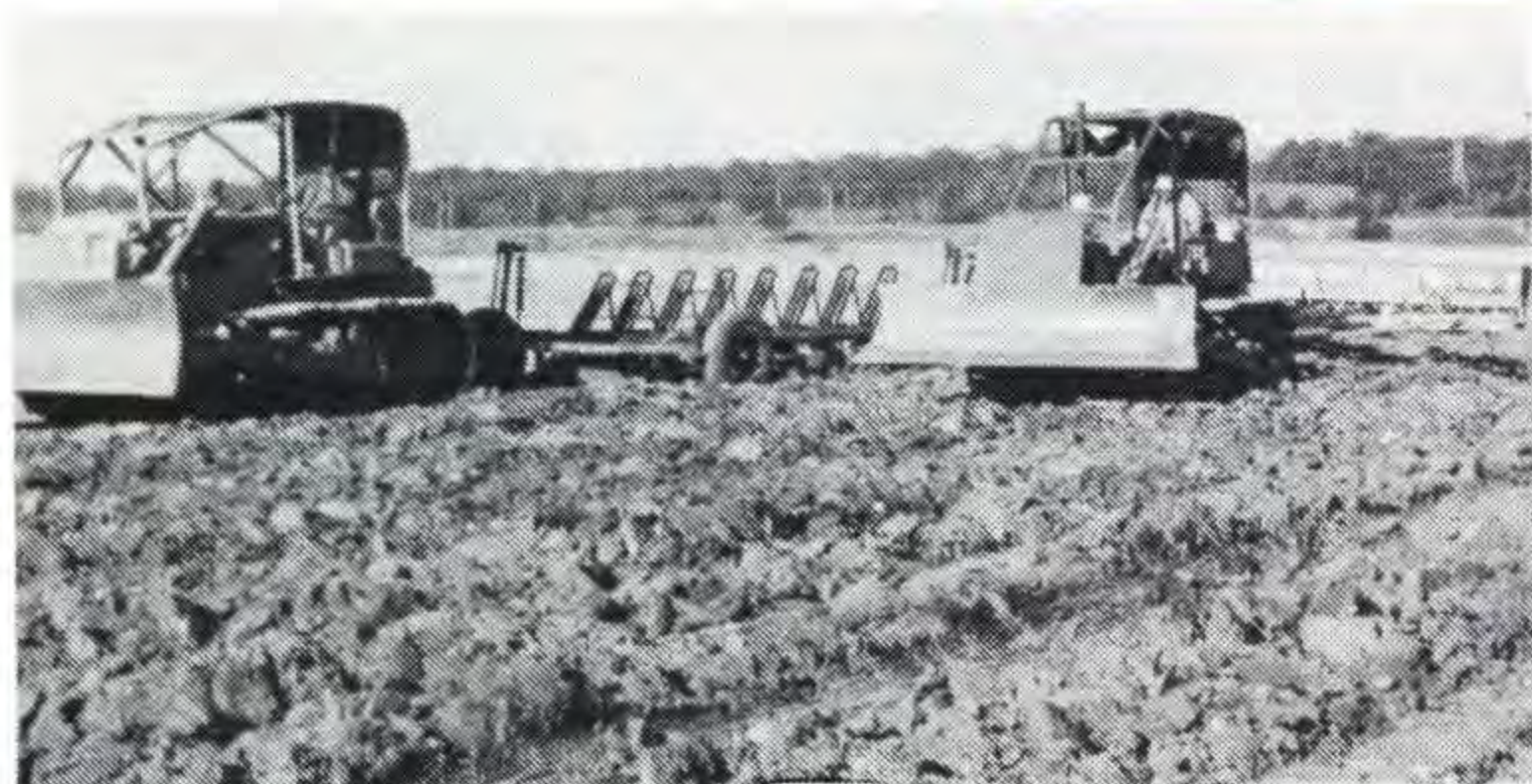
CONTACT' photographer took this picture of the two bulldozers busy at work recently.
