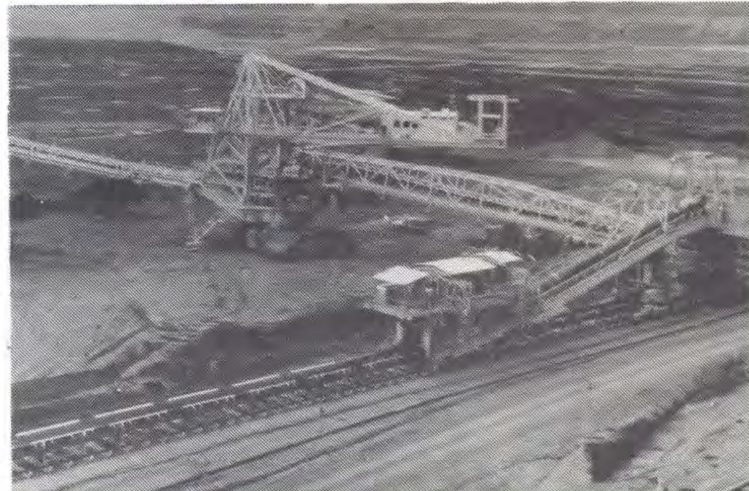
TS3 is pictured busy at work spreading overburden onto the new overburden dump in the southern corner of the Yallourn open cut.
