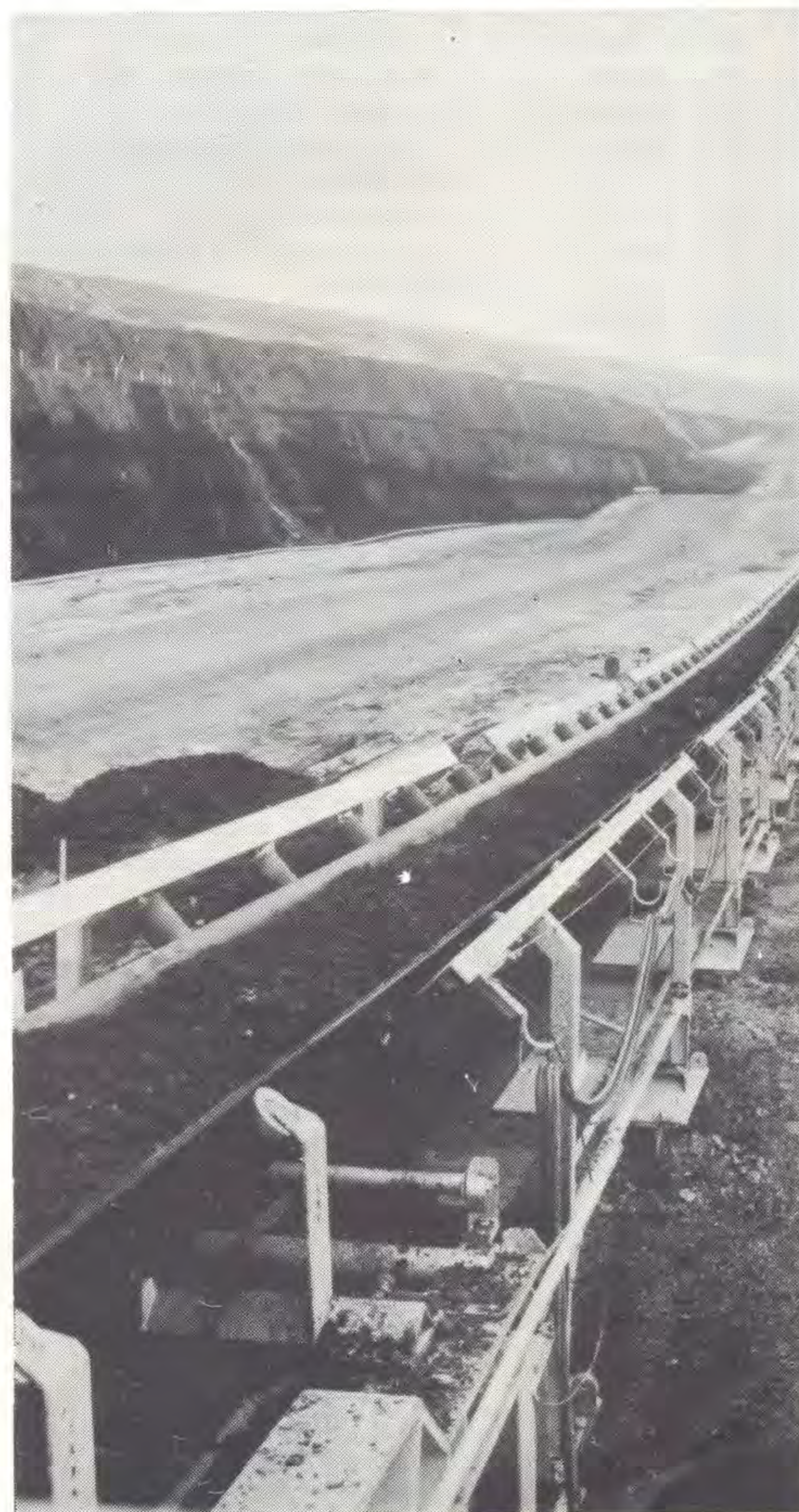
No. 13 overburden dredger feeds the overburden onto the new conveyor system in the Yallourn open cut.
