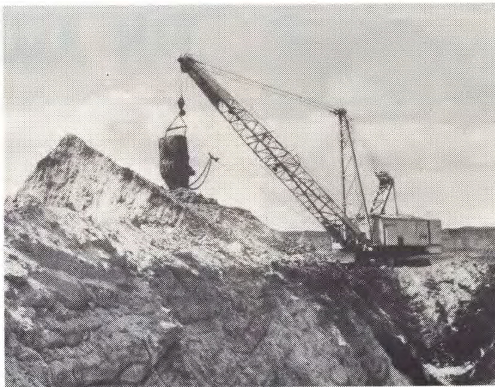
The former Yallourn North extension dragline is pictured digging at the clayhole site in the Morwell open cut.
