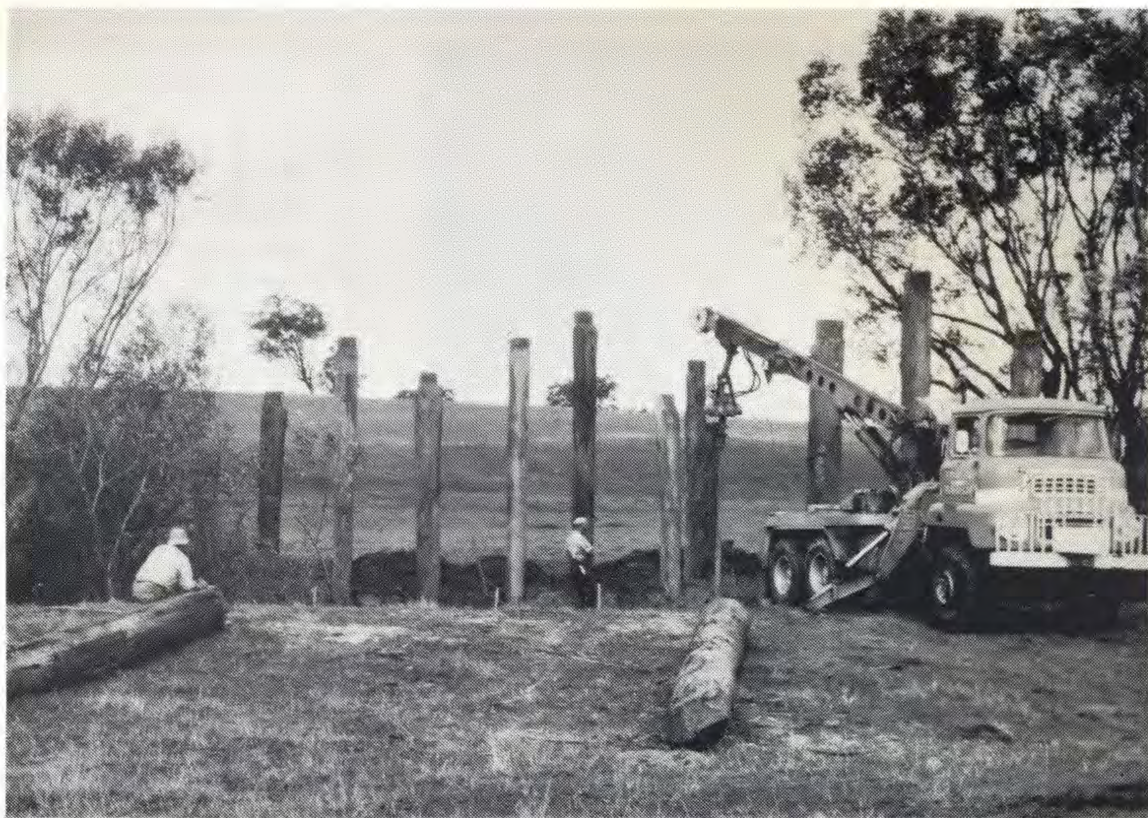
Contractors (above) were busy at work early this month constructing a temporary bridge at Traralgon South Creek.
