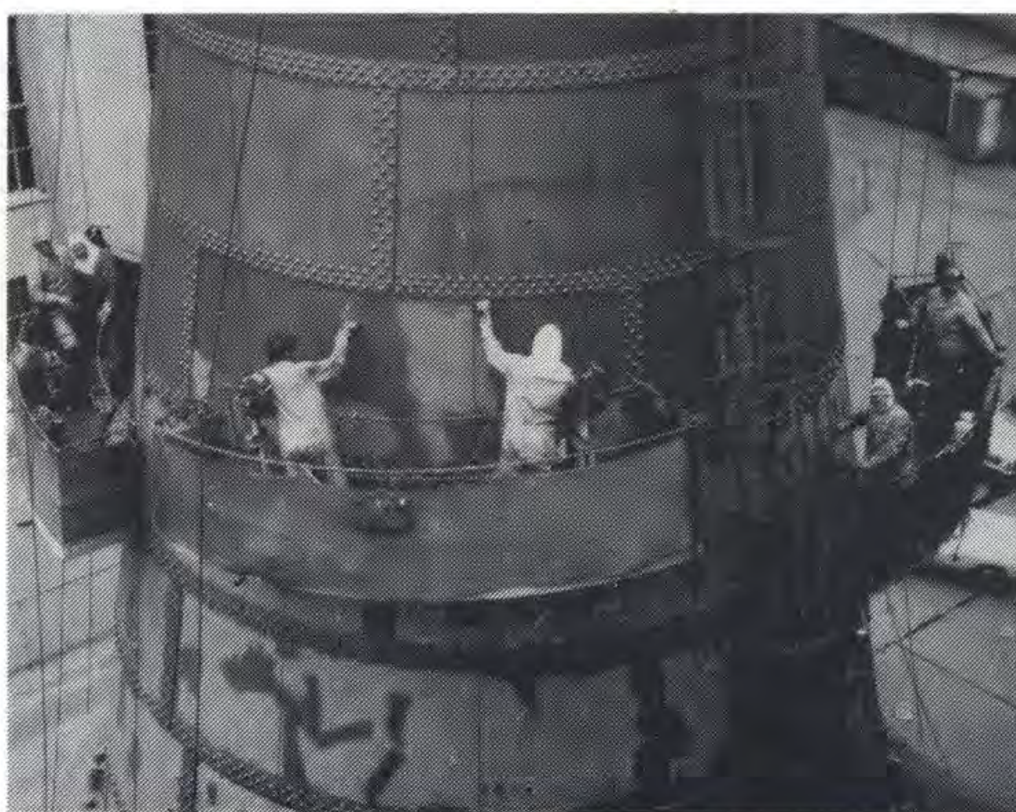
Busy at work painting the the briquette factory chimney are six of the painters.
