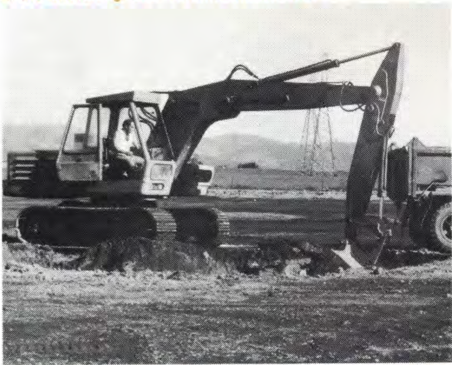
Above: This large back-hoe excavates a hole on the gas turbine site near the Hazelwood 500KV switchyard.
