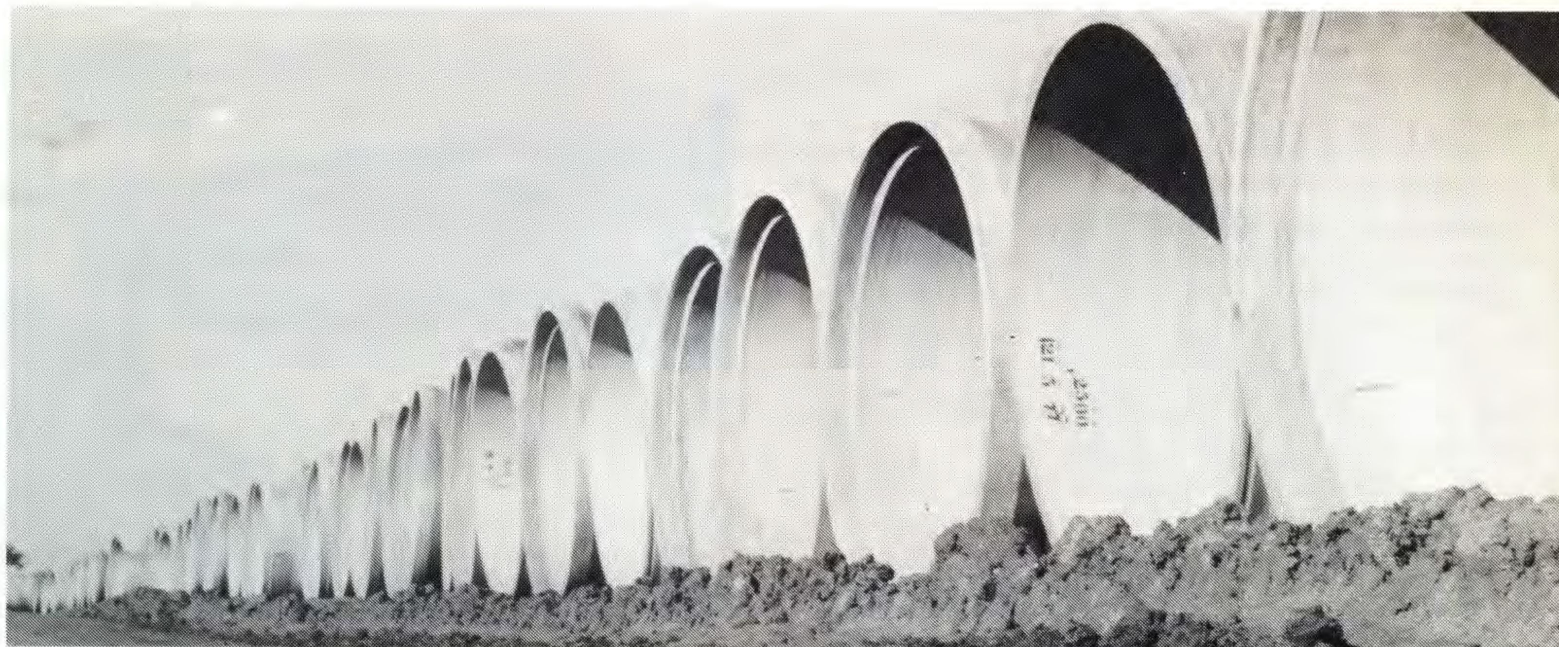
Some of the 1,500, five tonne, pipes to be used as part of the main drainage from the power station and the coal storage area are pictured above.
