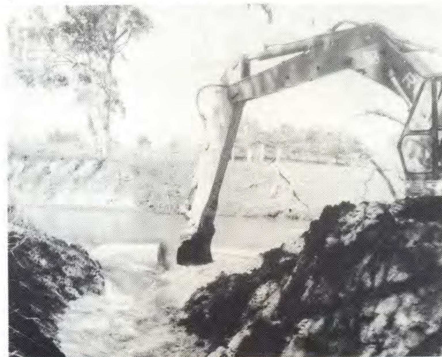
A back-hoe was used to dig through the earth embankment to allow the Morwell River to flow through the new diversion channel.
