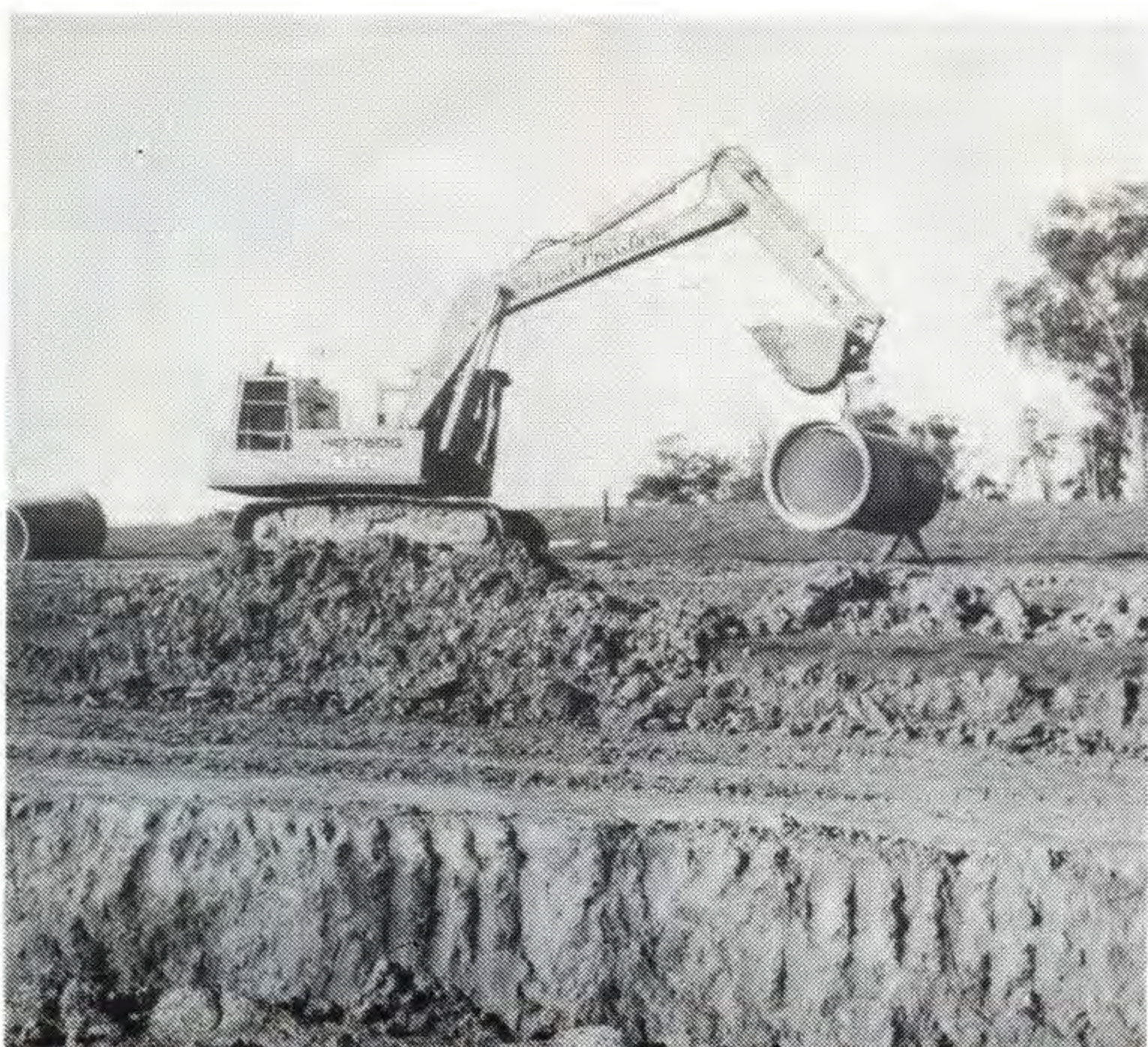
A number of smaller pipes are placed into position by a back-hoe as the picture above indicates.
