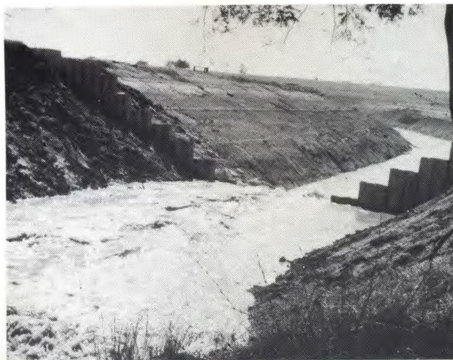
The first water to flow through the new Morwell River Diversion channel is pictured above.
