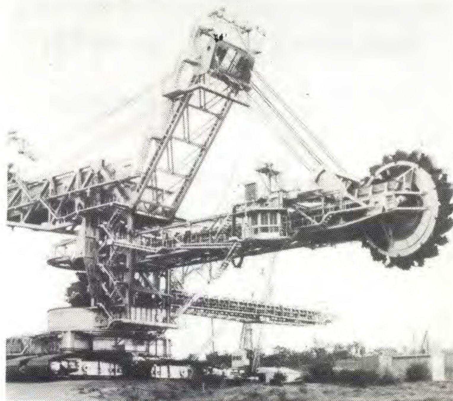
No. 13 dredger is pictured (right) during its commissioning tests at Hernes Oak early this month.
