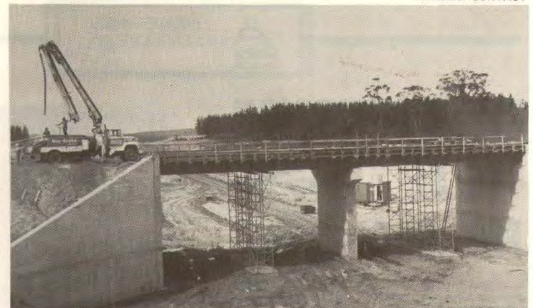
Work on the Barton's Lane overpass was nearing completion when this picture was taken
