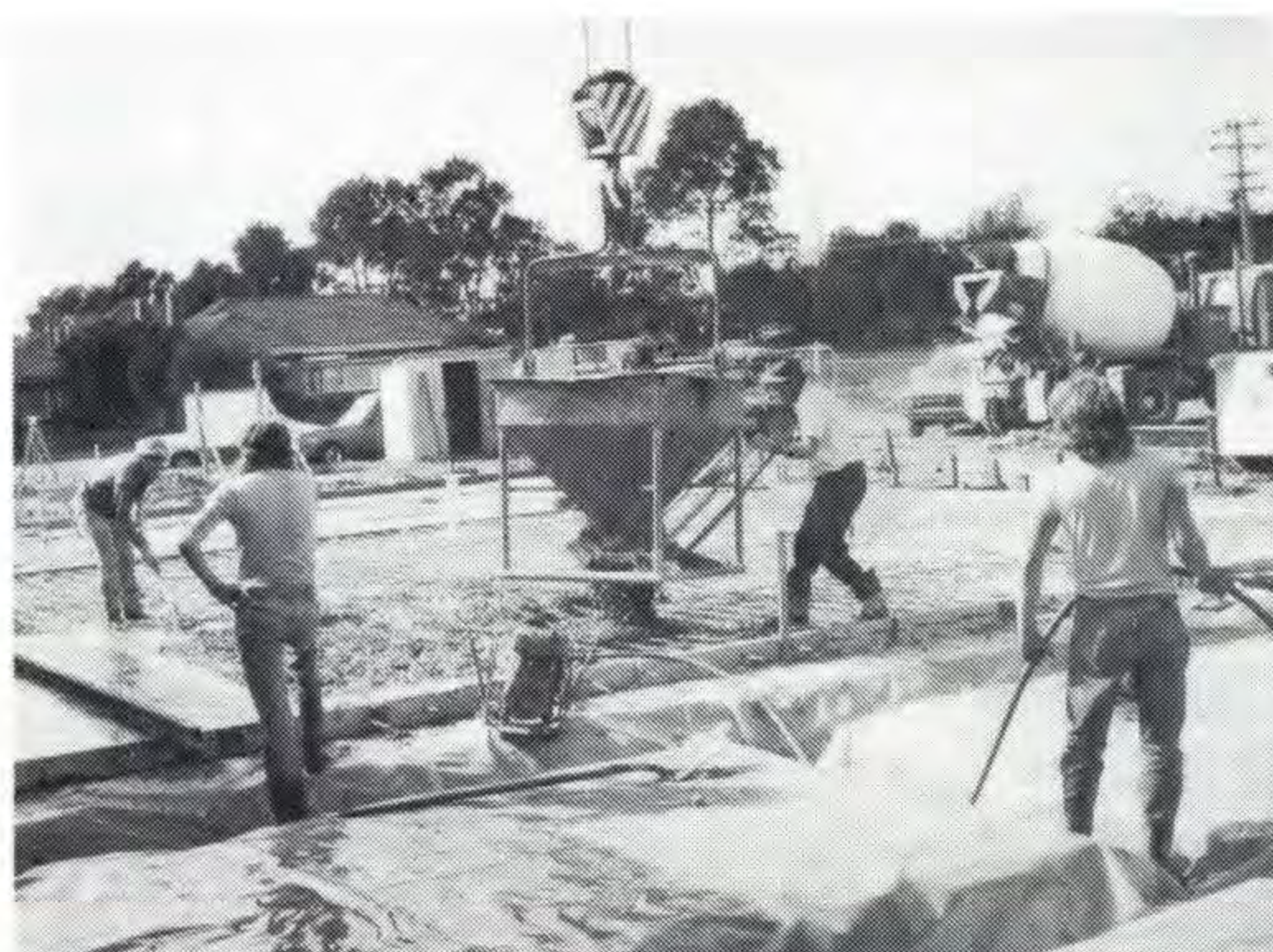
Foundation works for the new bowling club extensions were in full swing when CONTACT visited the site early this month.
