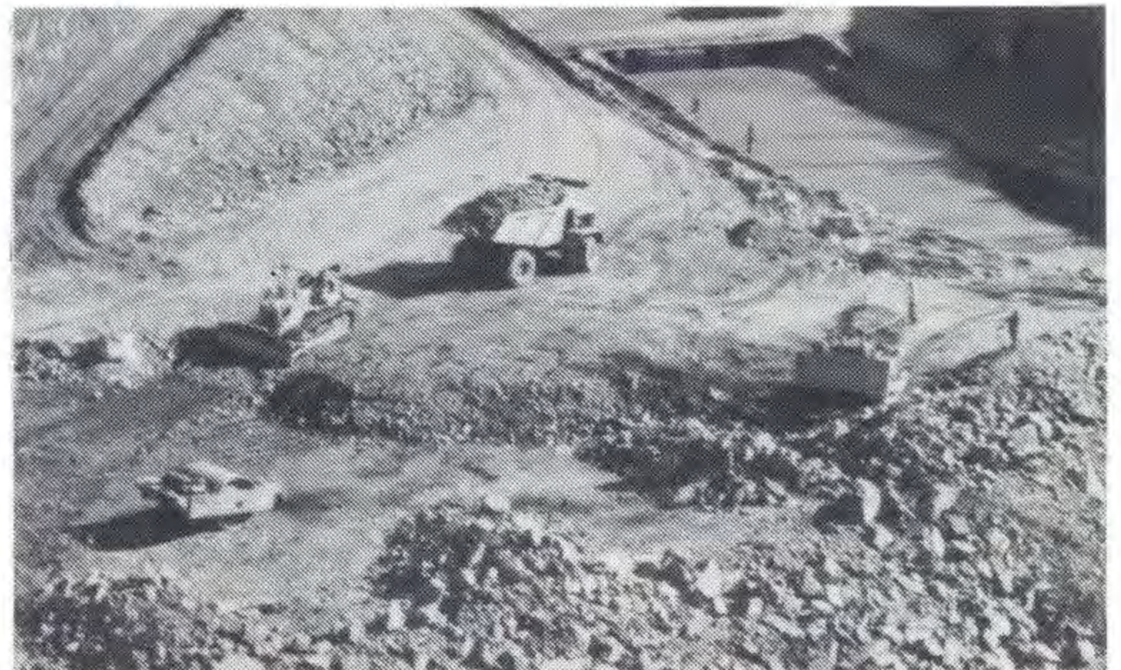
Heavy earth-moving equipment is involved in the massive operation of preparing the site for the dam wall construction.
