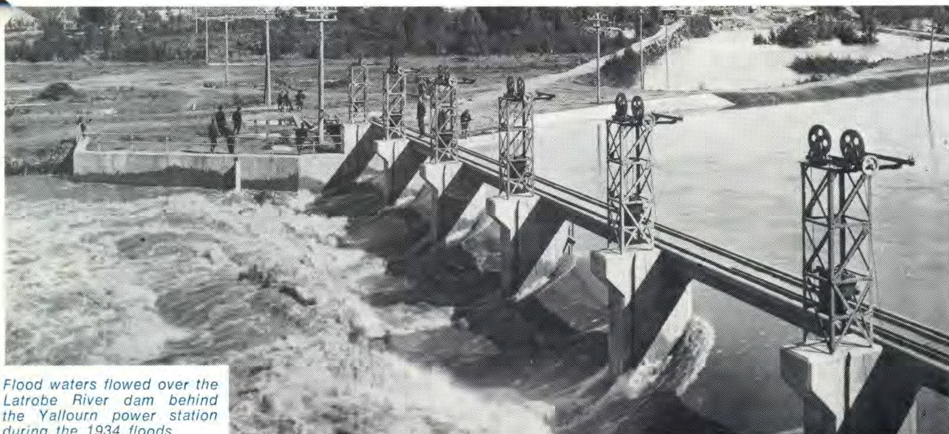
The Latrobe River bridge (left) on the Yallourn North road was closed for a period due to the floods.
