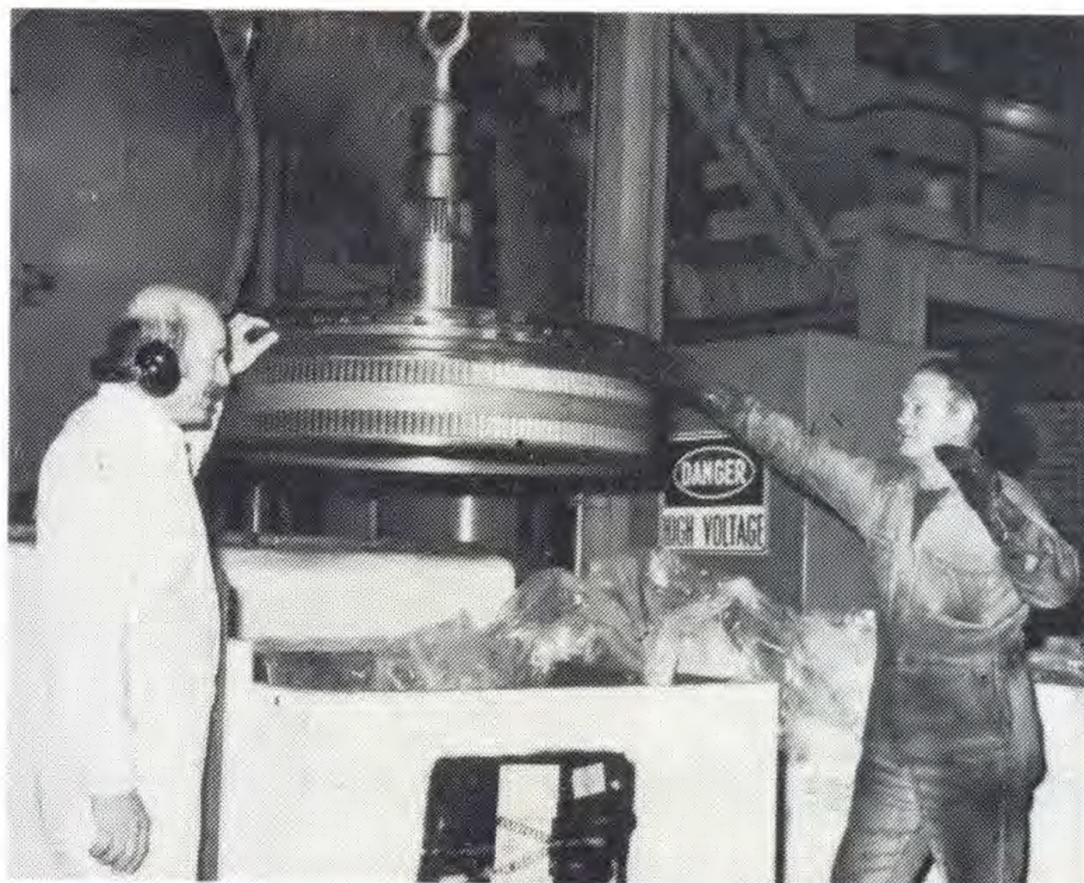
Unloading the turbine rotor was carried out by Overseer Tom Amalos (left) and Ted Rockall (rigger).
