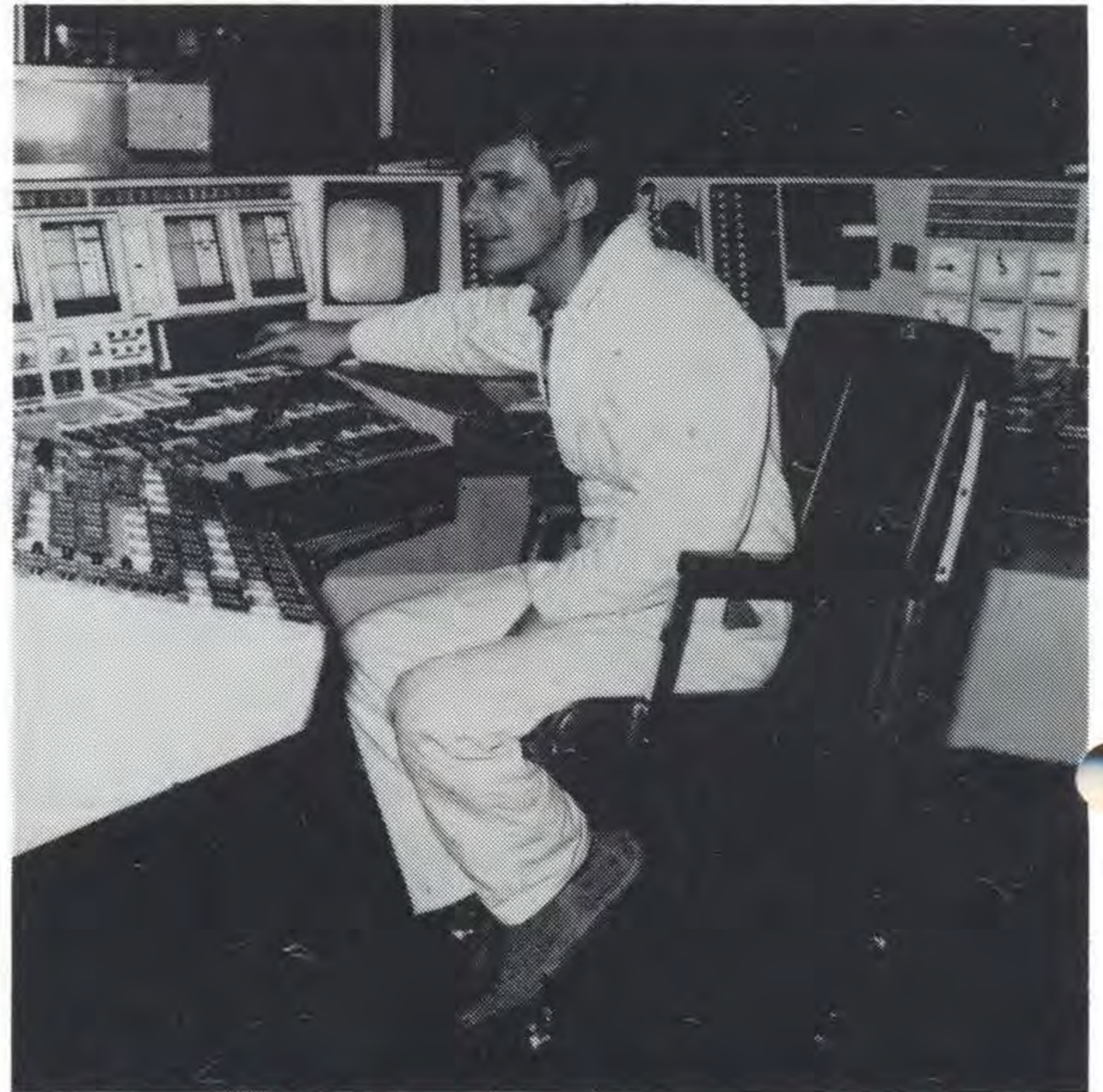
Unit controller Ray Roberts of Churchill was pictured by CONTACT's photographer in one of the Hazelwood power station's control rooms which is similar to the new simulator.
