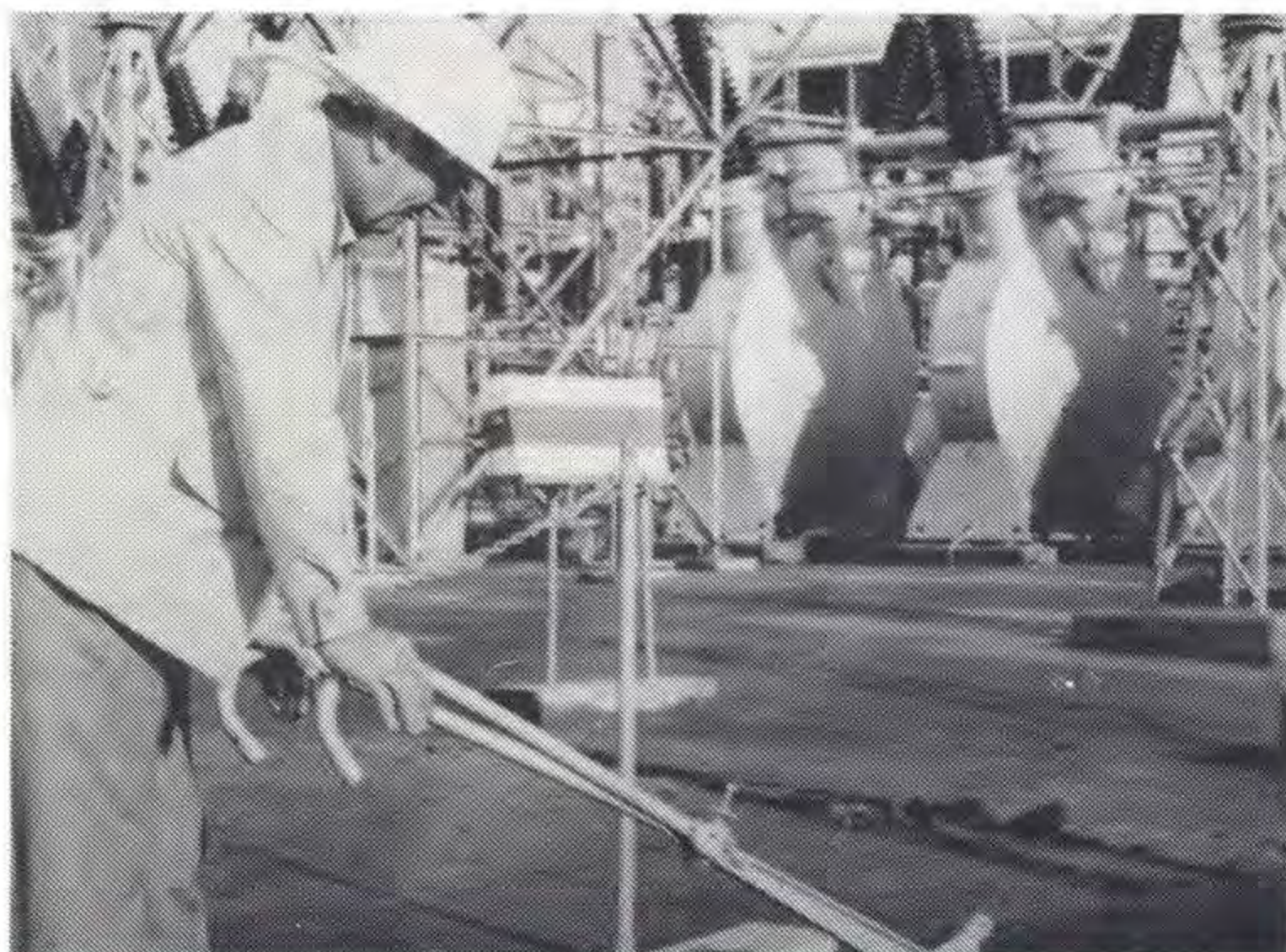
Fred Barnes demonstrated his invention outside the Yallourn power station switchyard early this month.
