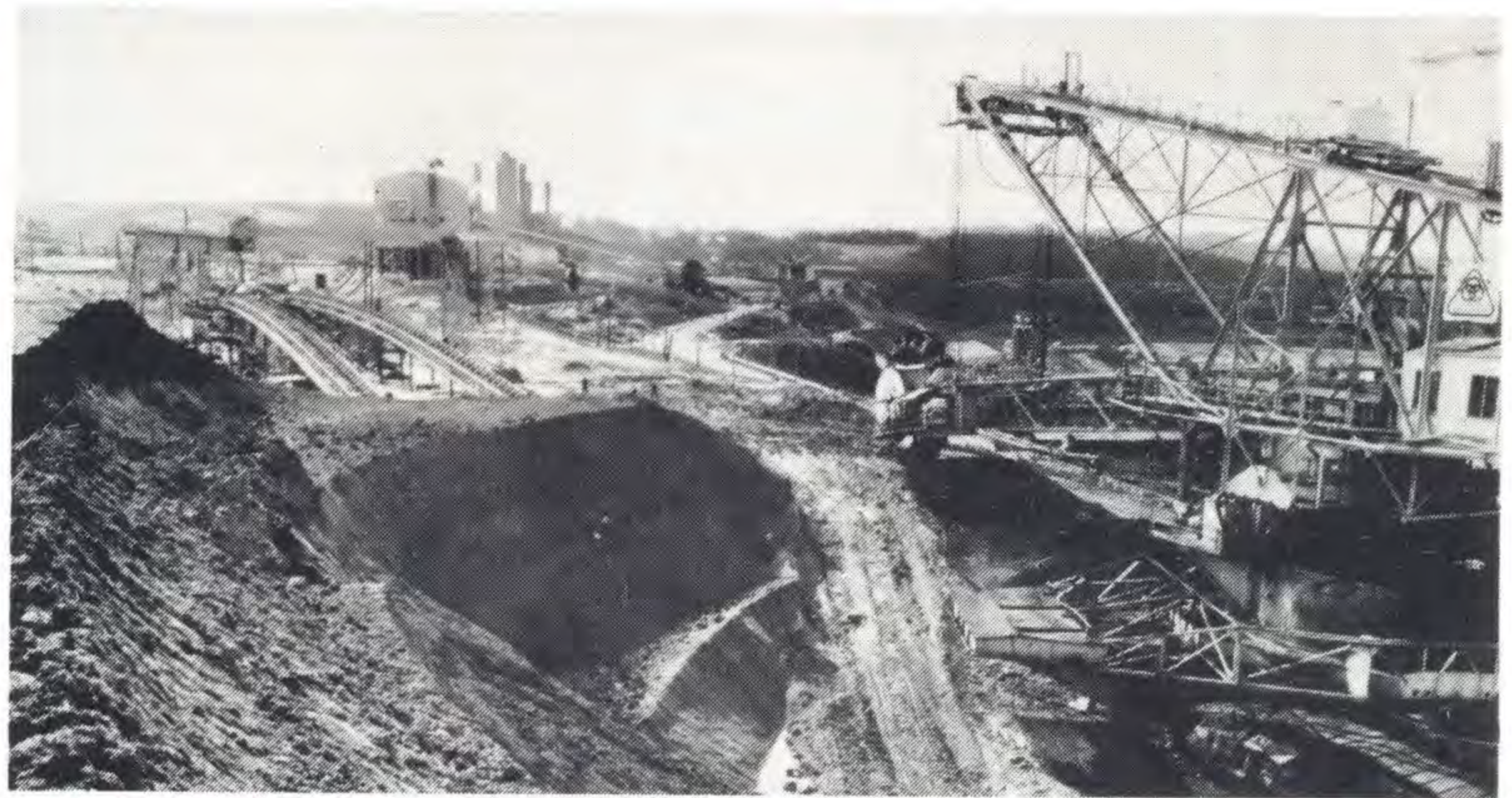
No. 7 dredger (above) eats its way through the Bulge. Yallourn power station is picture in the background.
