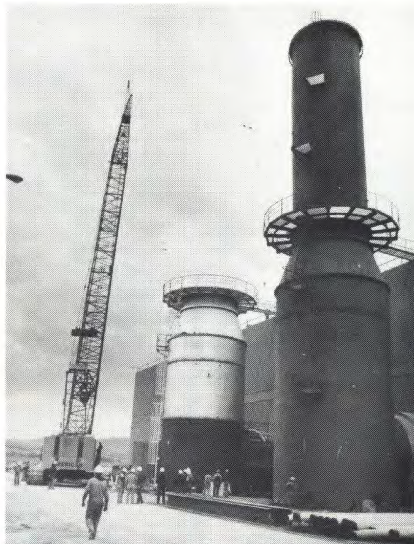
The huge 200 tonne crane makes the Unit 2 chimney at Jeeralang Gas Turbine station look like a dwarf.
