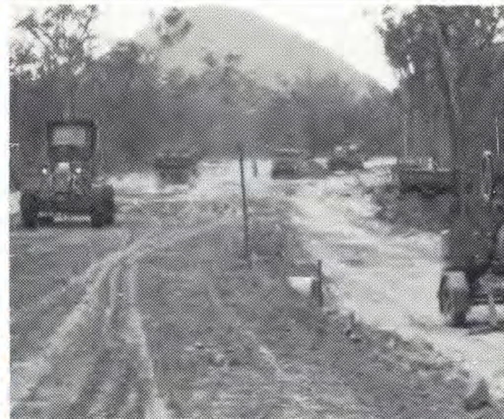
LEFT: Heavy earth moving equipment preparing roads for next year's NATO exercise.
