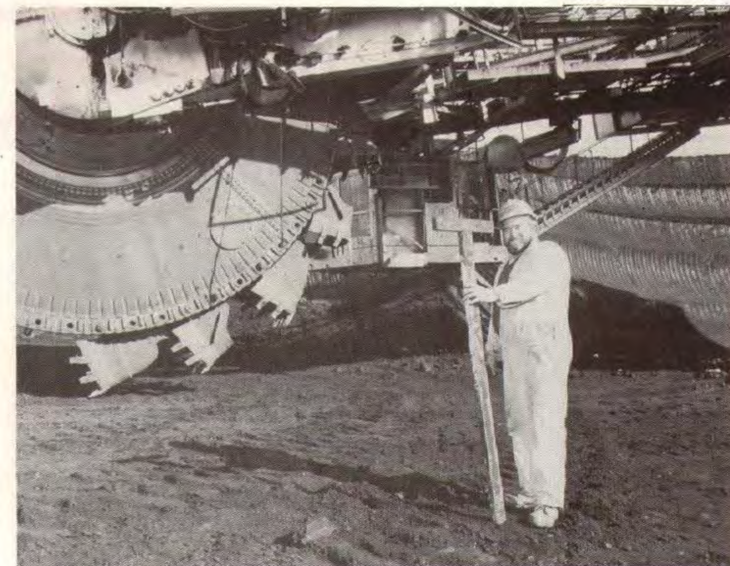
ABOVE: A member of the No. 9 dredger crew, bedman Dick Griffiths of Morwell.
