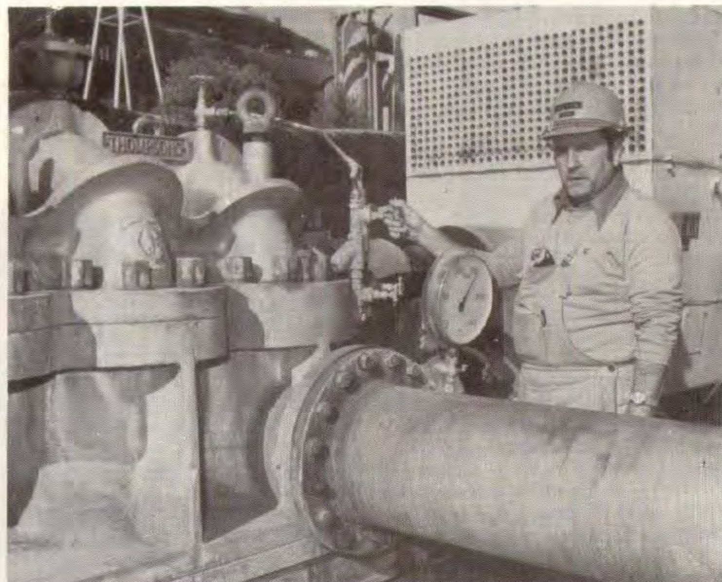
BELOW: Pumpman Kevin Durea of Morwell checks pressure levels of the pumps in the Morwell open cut.
