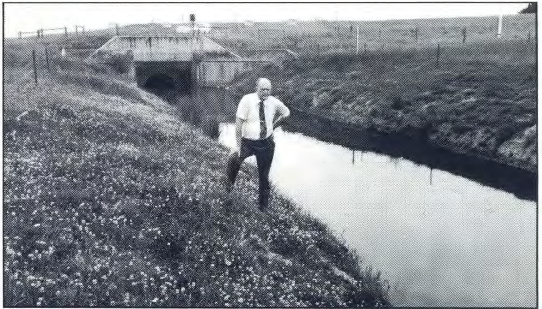
Above: The Morwell River diversion with Ian McDonald in the foreground. The tunnel the river is entering continues for three kilometres.
