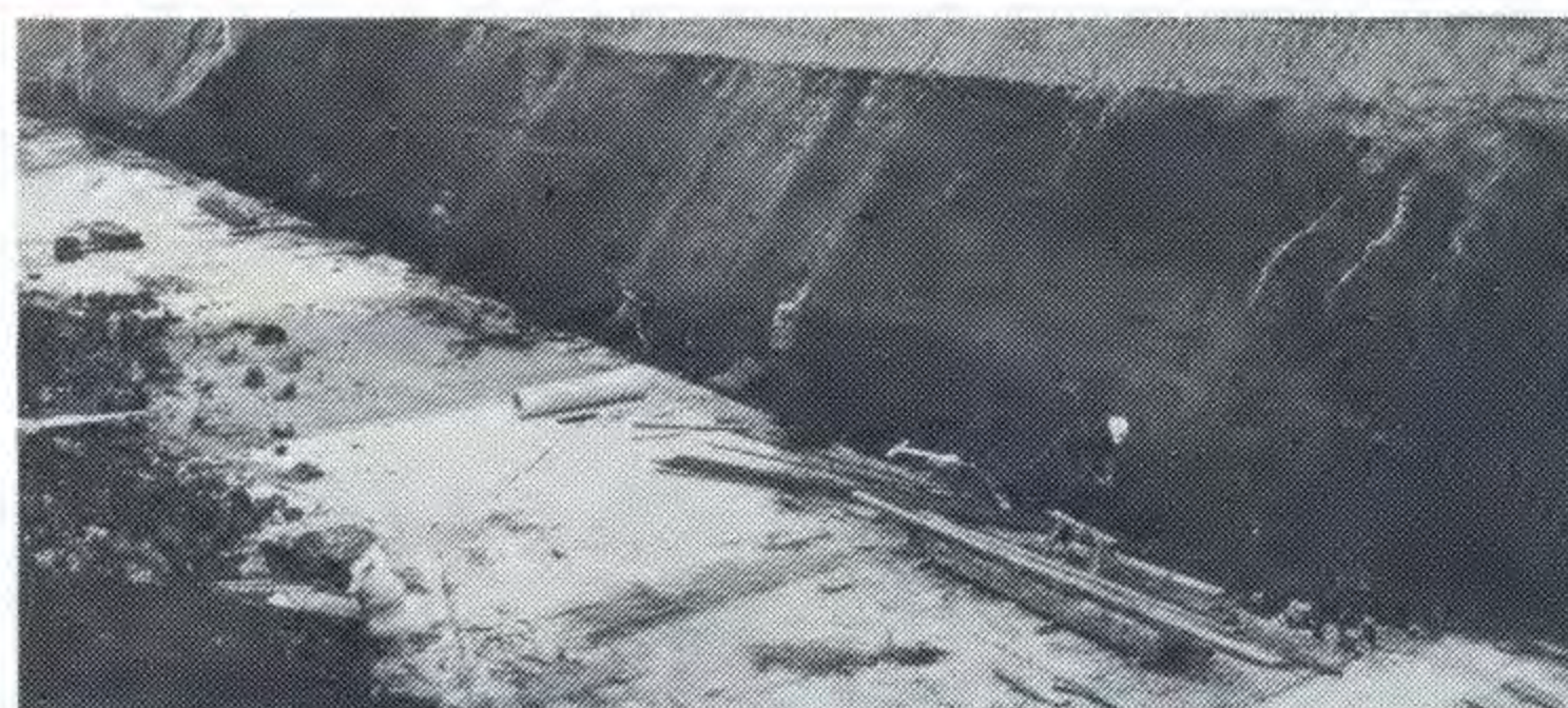
Above: The extended slab of number 11 ditch bunker.
