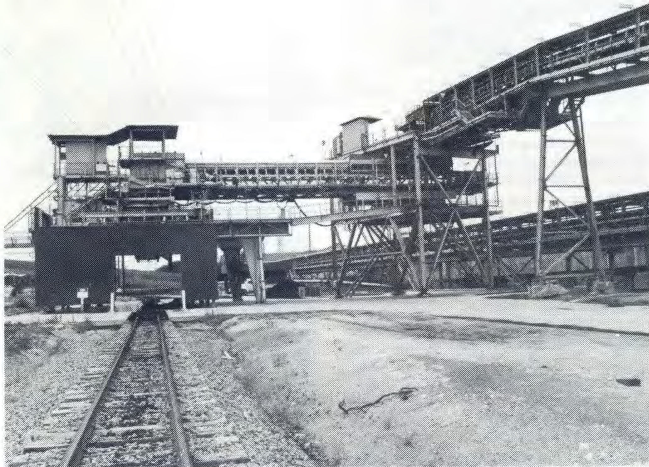
Above: The new Yallourn coal loading station showing the new bridge section. The station used to be part of the number 12 conveyor system.
