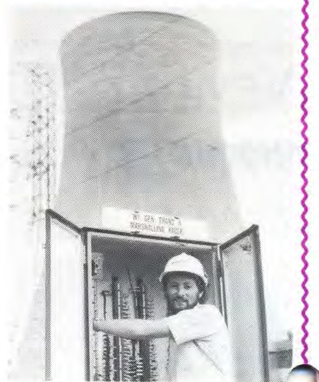
Ian is pictured testing the electrical wiring around W Station.
