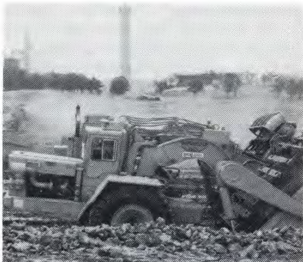
Above: Some of the scrapers excavating and placing select fill.
