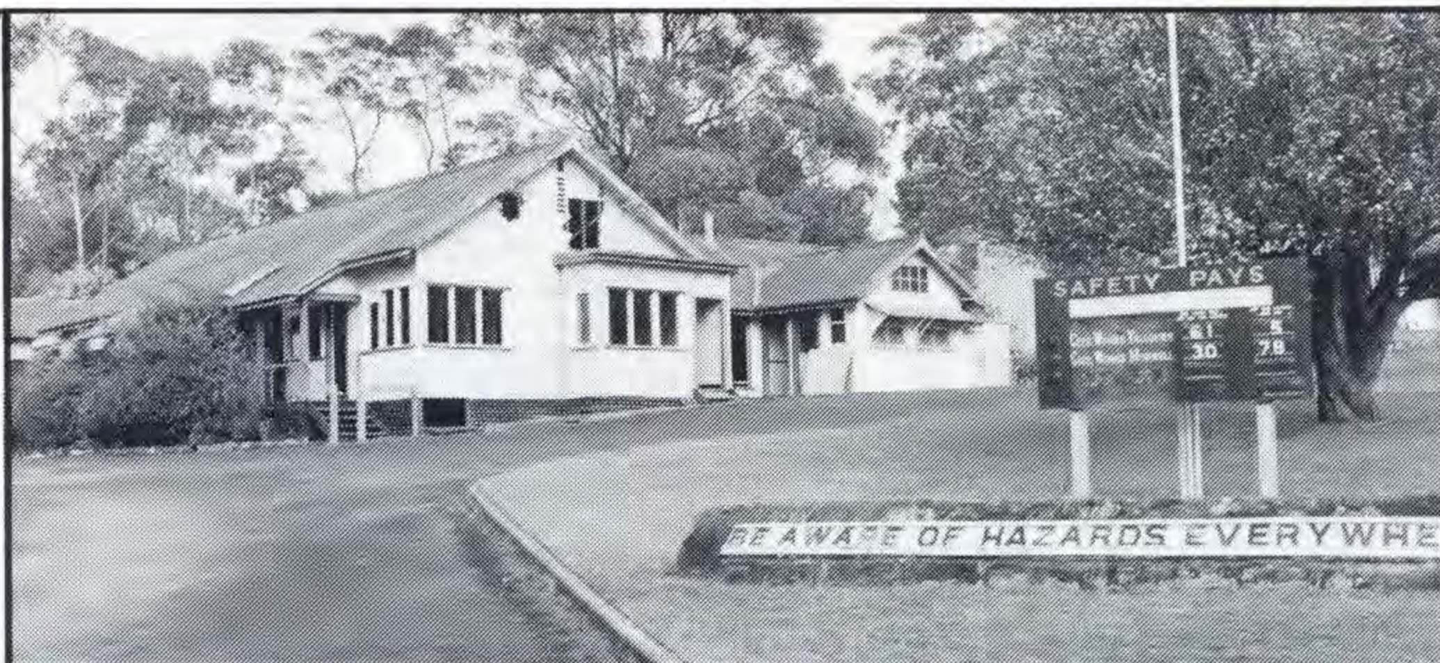
Above: The old municipal offices in Yallourn — as they once were.
