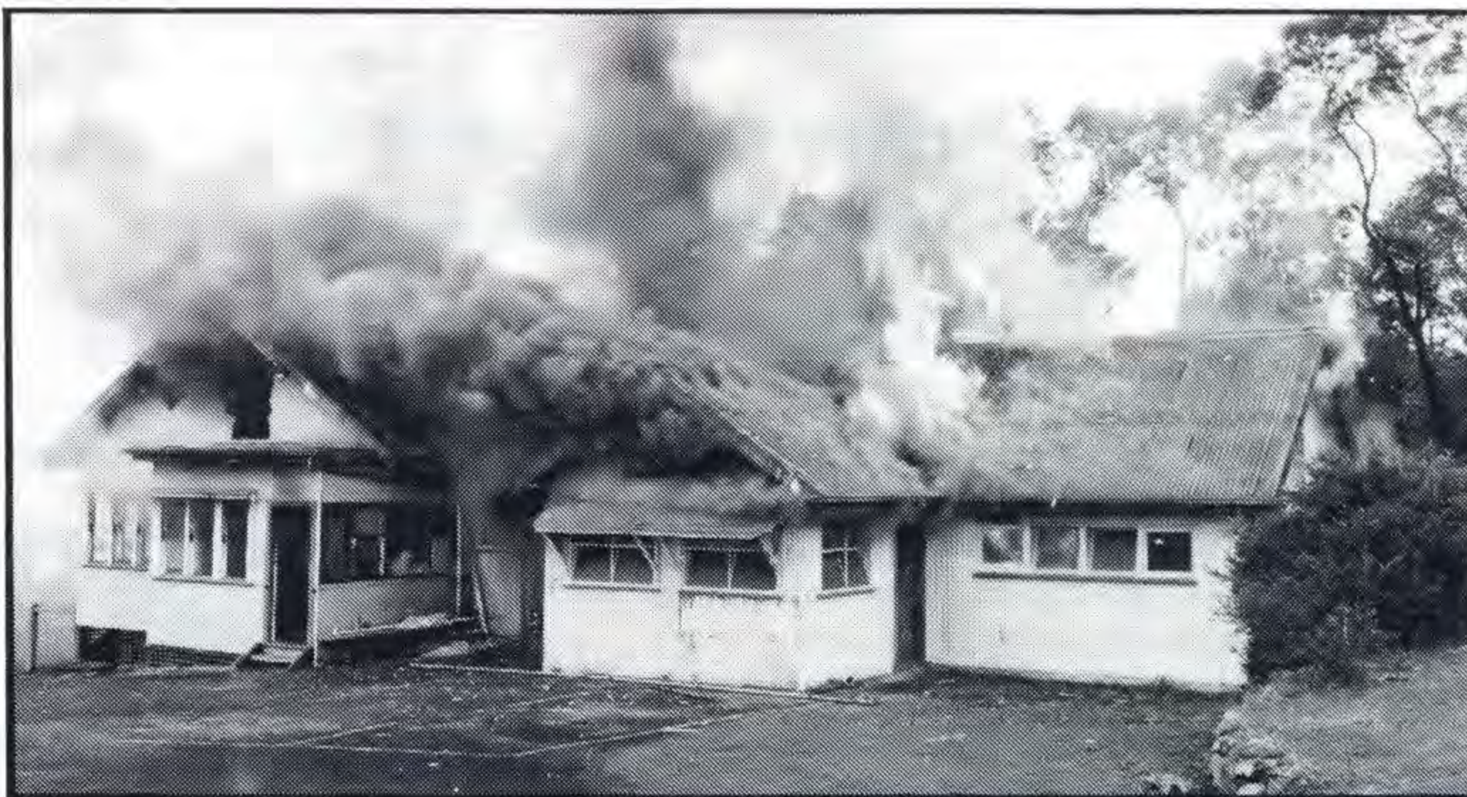
Above: At the height of the fire, pieces of exploded asbestos cement sheeting can be seen littering the ground.
