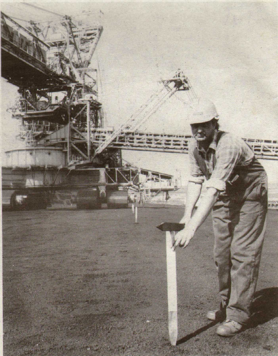
Everyone at Yallourn Open Cut is treating health and safety seriously. For the first time in history, YOC, has recorded a month with no LTI's and no one on long term Workcover. Dredger driver Paul Gridley putting pegs into the ground to mark the line for the dredger to follow.
