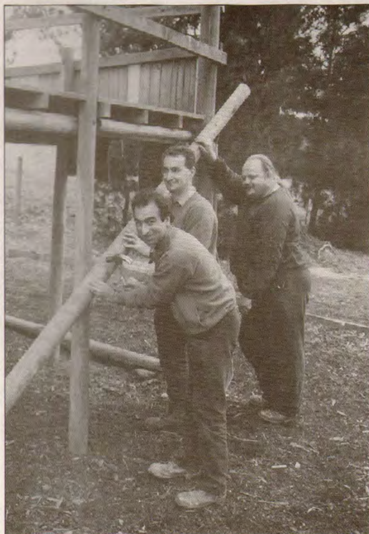
Paul Dimos, Greg Curtis and John Hughes replacing playground equipment at Yinnar South Primary School.
