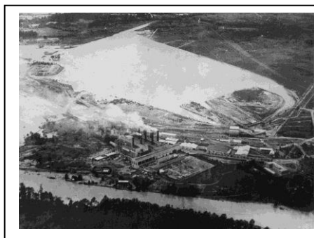
Aerial View of Open Cut before & after 1934 flood. 4000 million gallons of water were pumped out over 4 1/2 months.
