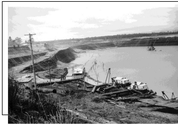
Open Cut during flood, showing pipes in the foreground for pumping.
