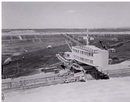
A dredge in the open-cut
