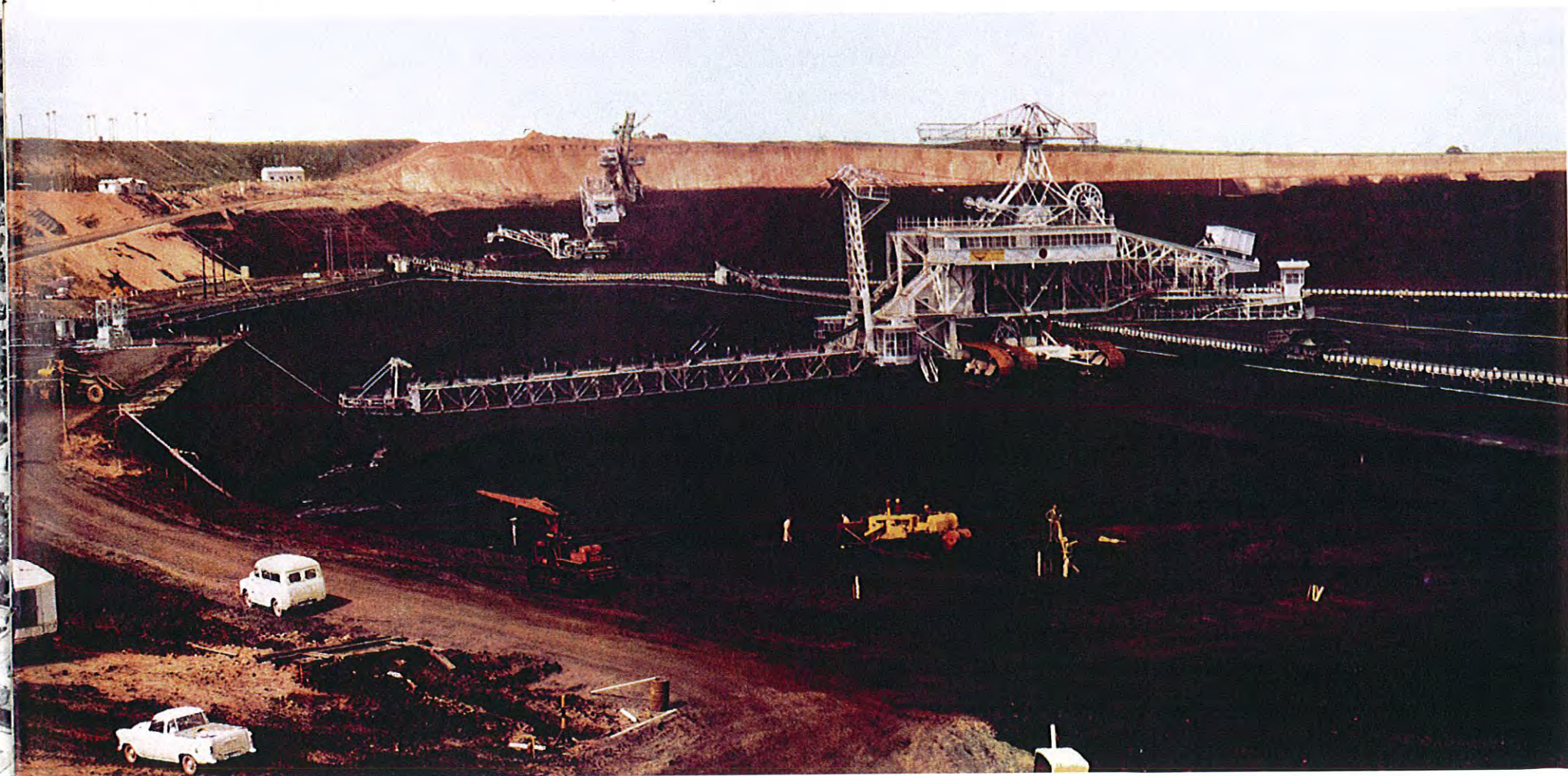
Morwell Open Cut
