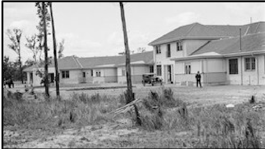
December 1928 at the Yallourn Hospital construction site. Source: State Library of Victoria. Reference: H2009.18/248.
