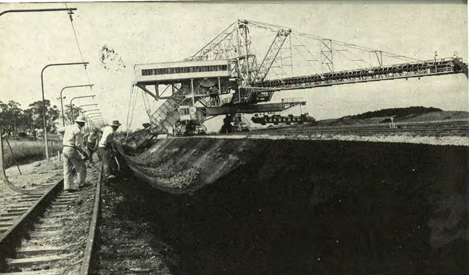
Trains dump their loads of overburden in this ditch. The men keep the lines clear, and the spreader distributes the loads.
