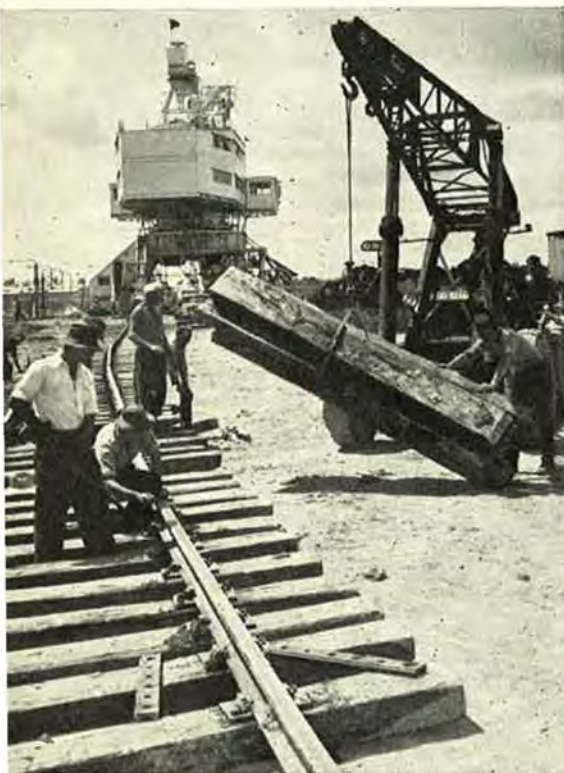
Many kinds of railway sleepers are prepared at Morwell. Here a crane brings in more for a temporary line to move the dredger in the background, flying the nautical Blue Peter.
