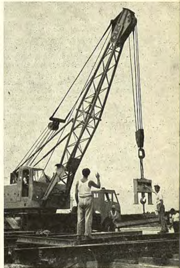
This crane weighs as it lifts steelwork for the contractors. L. to R. W. Harris, J. Rousws (Greece), Frank Rowin, Andre Hedl (Hungary), and the waiting crane-driver is Ken Brownbill.
