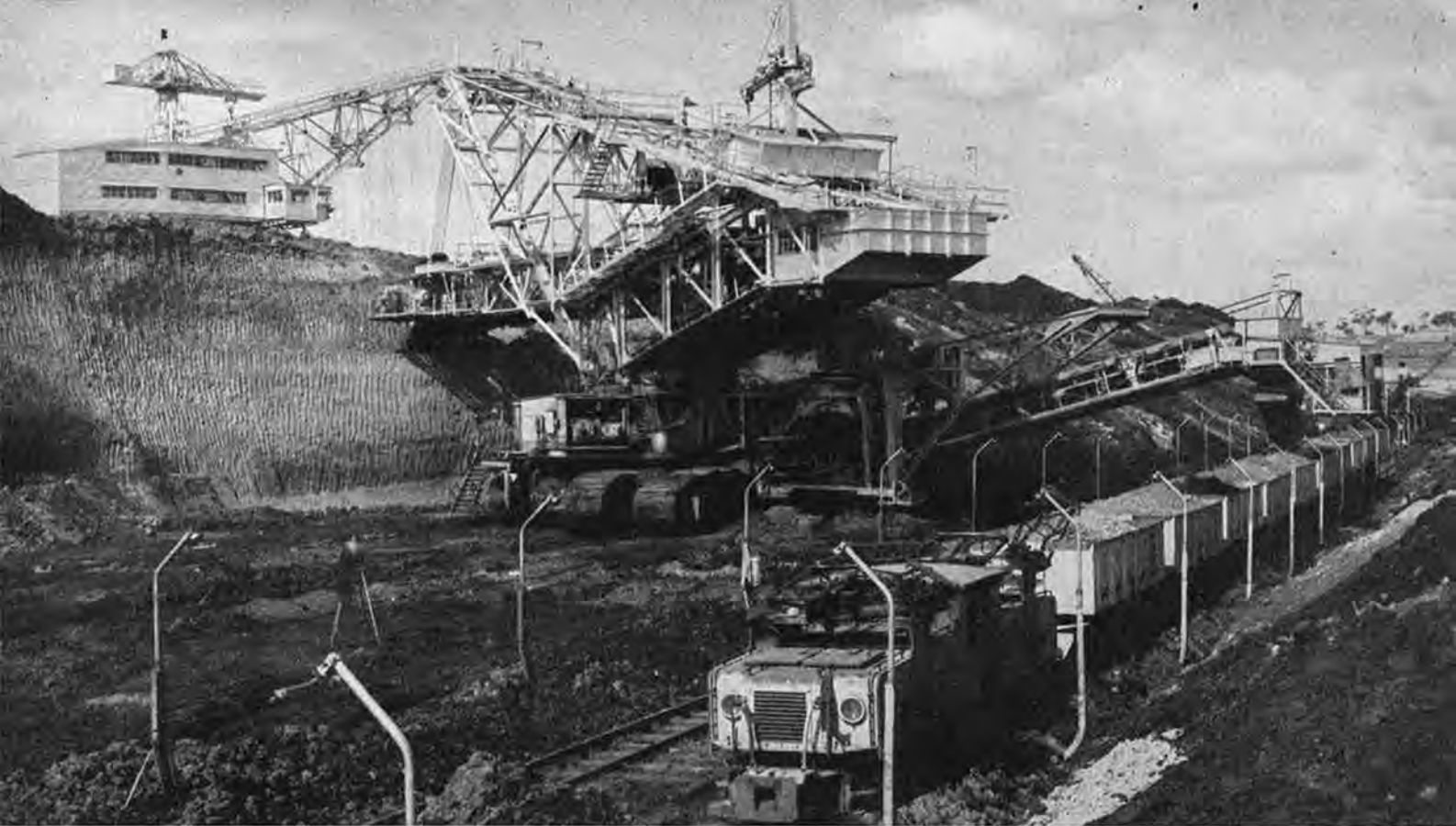
One dredger digs out overburden and fills the waiting train in open cut. Another waits on top to move to its working point.
