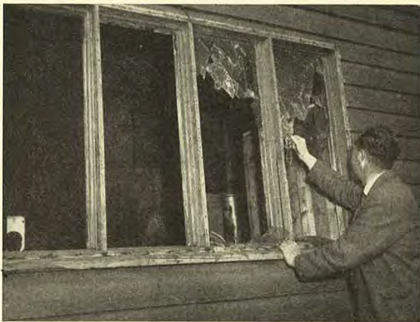
The winter gales could blow through this dressing room window for all wreckers care. Determination was needed to break the wire-reinforced glass.
