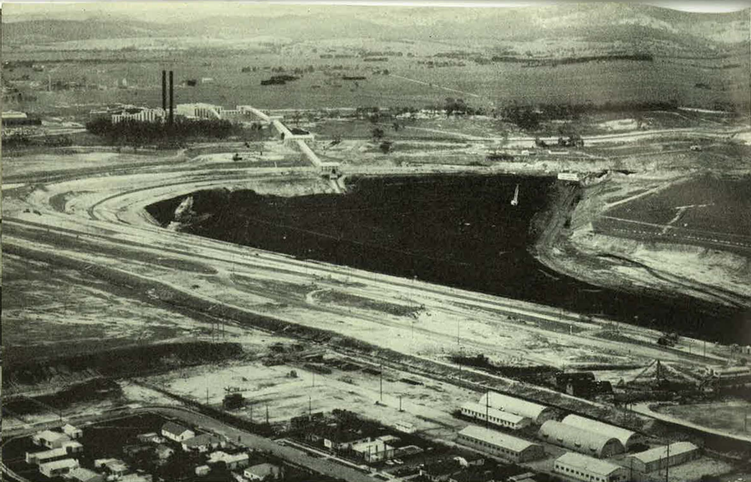
AT THE NEW MORWELL OPEN CUT , which is being developed to supply brown coal for the Morwell power station and briquette factories, more than two million cubic yards of over-
