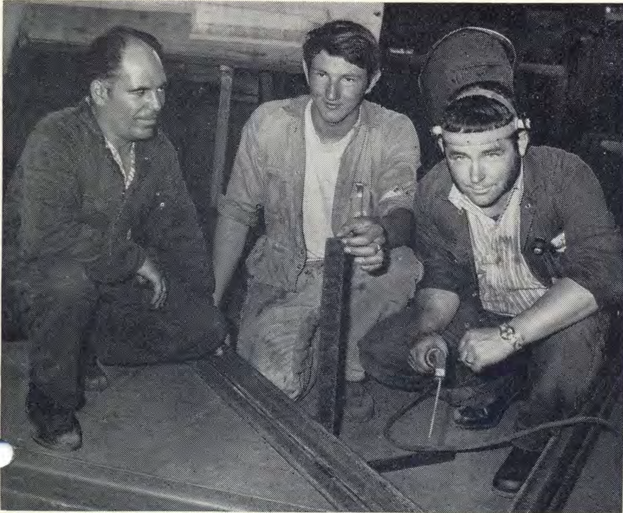
Preparing steelwork in the shop for a new insert for a conveyor boom are (l. to r.) Charlie Farrugia, Victor Salienko and Roger Reeves.
