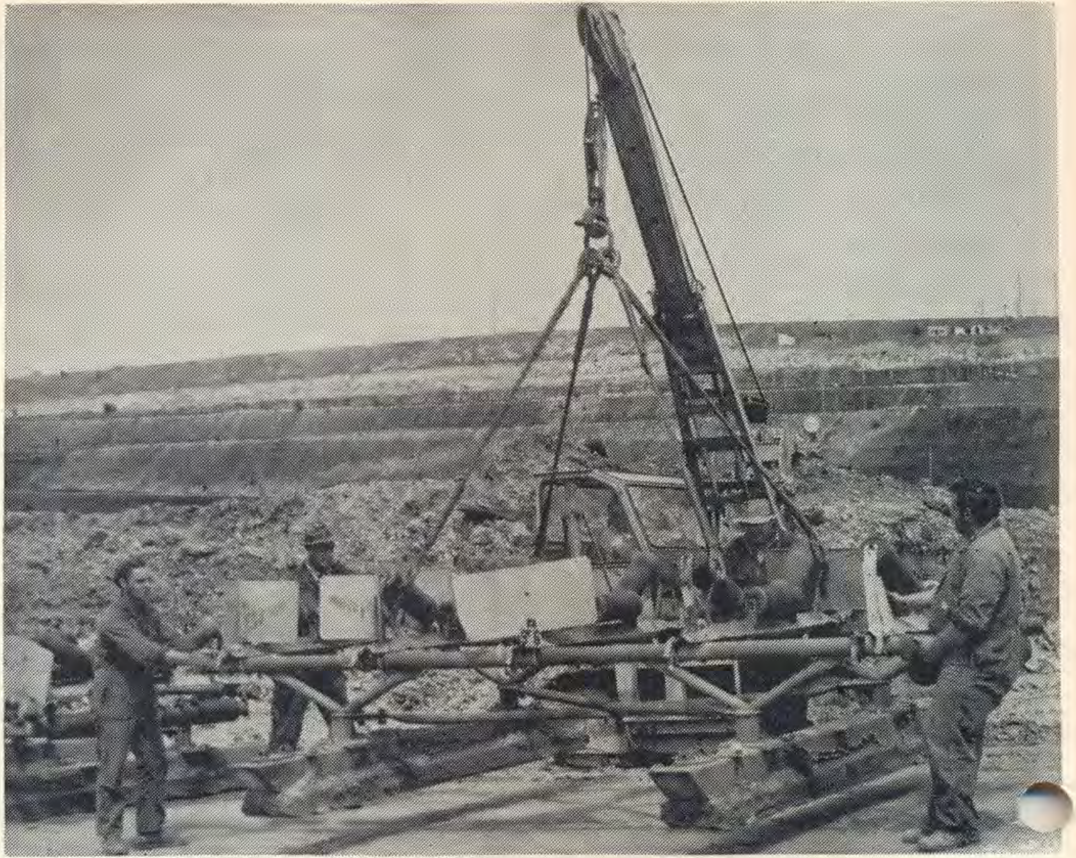
Peter Anderson, Laurie Campbell, Bill MacLean and Ron Deering, watched by crane driver Jack Richards, man oeuvre a section of a conveyor into position
